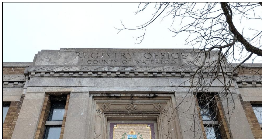
Photograph 1: Carved parapet stones above main entry
