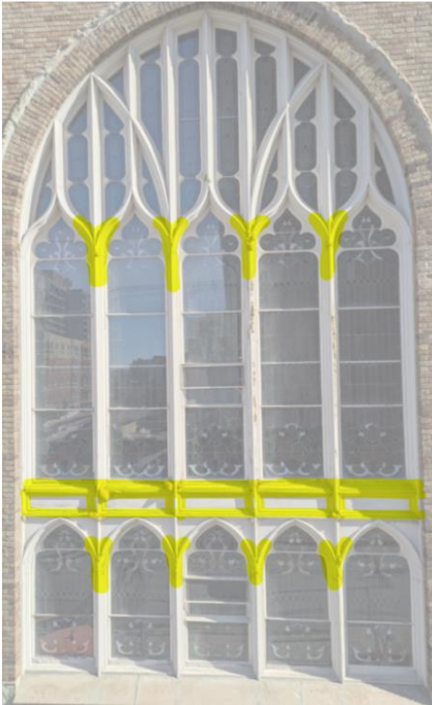
Figure 5.0 North Elevation (Benton St) – Wood Deterioration Highlighted in Yellow
