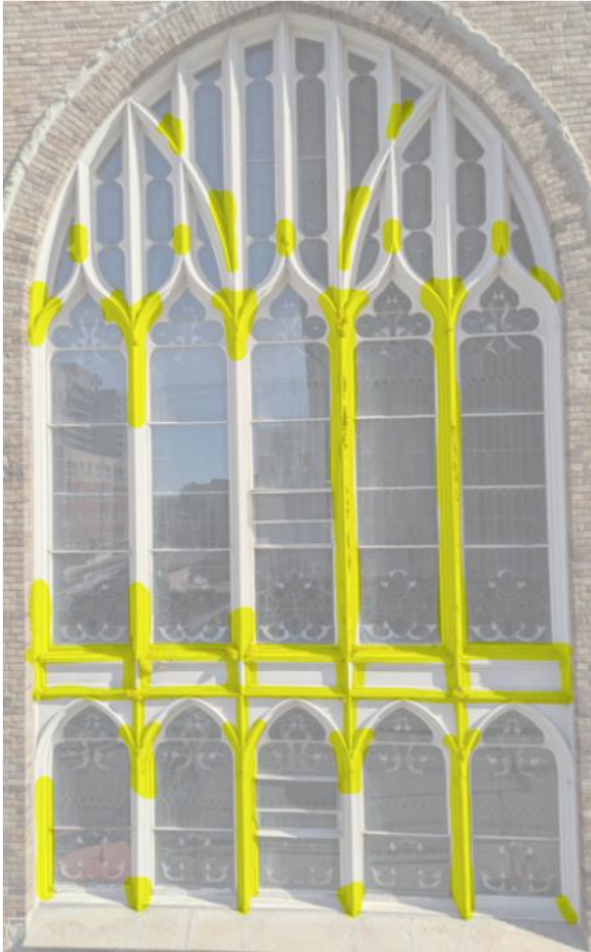
Figure 4.0 South Elevation (Church St) – Wood Deterioration Highlighted in Yellow
