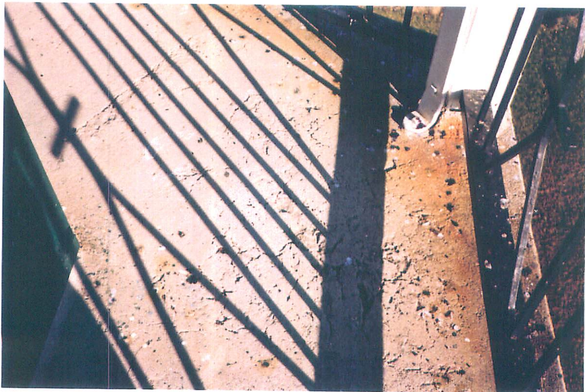
Photo 6: Top deck deterioration
