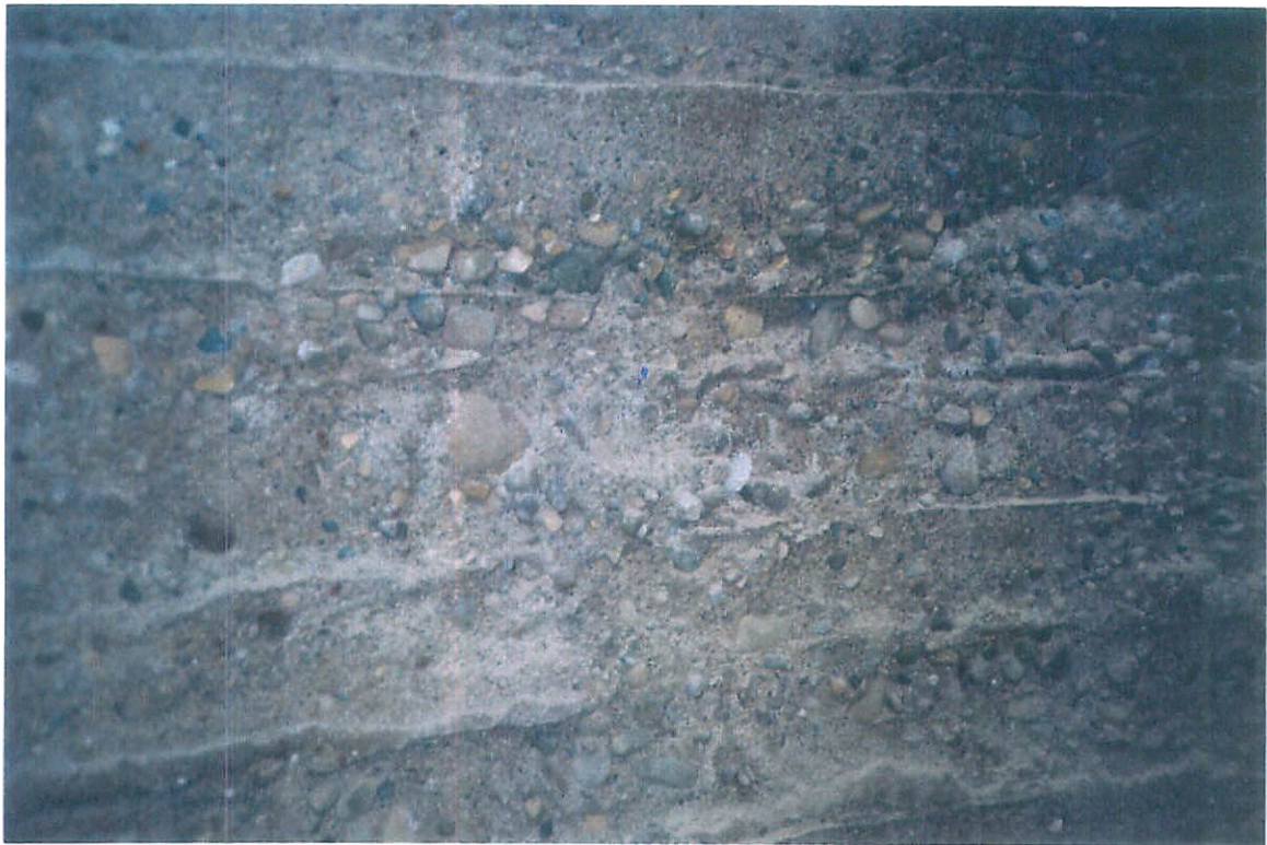
Photo 5: Interior concrete deterioration
