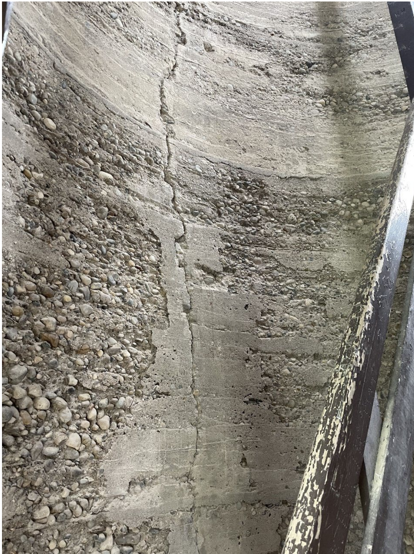
Figure 18: Example of crack in concrete interior of tower (A.S.I., 2024).
