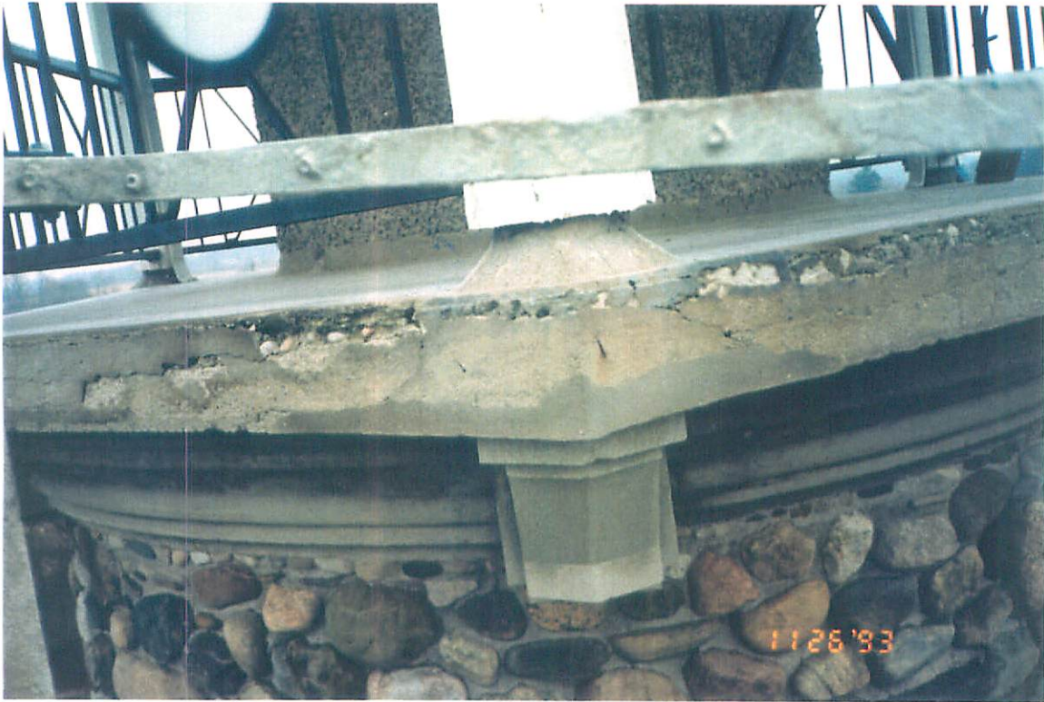
Photo 7: Top deck deterioration
