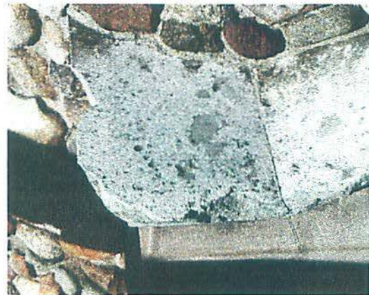
Gypsum crust on top of the entablature and chips of stone missing as a result of vandalism.
