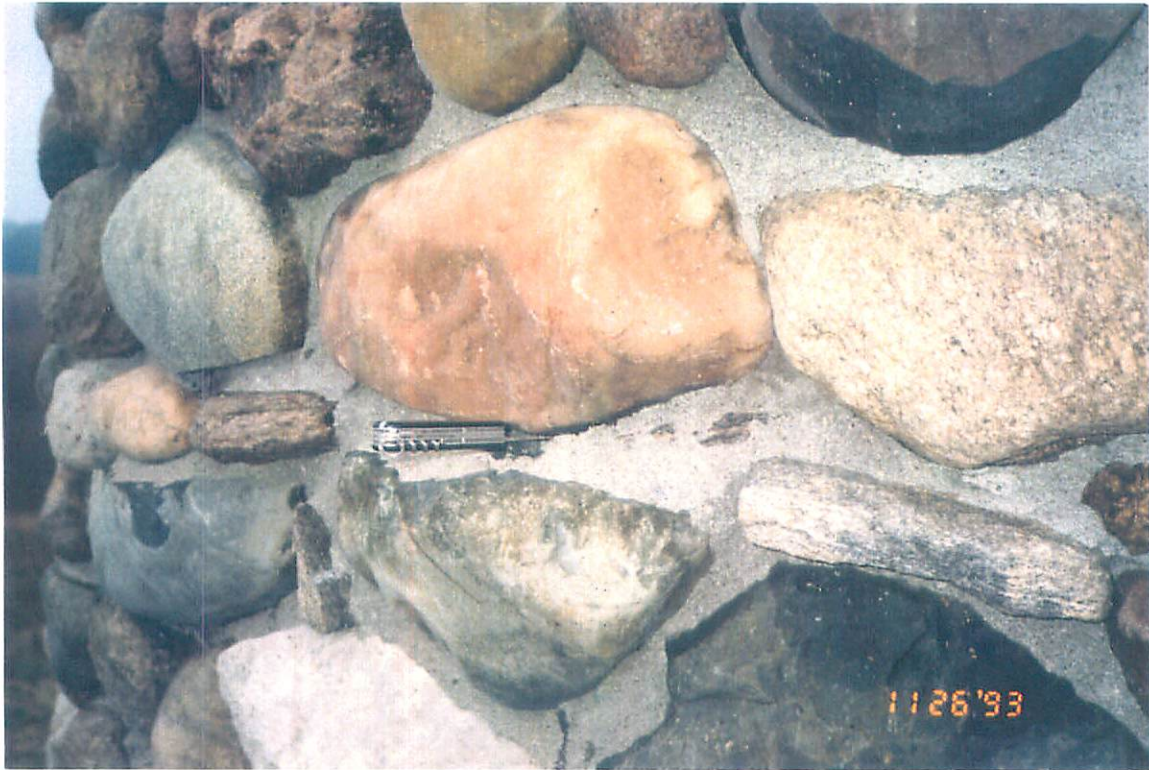
Photo 9: Stone joint deterioration
