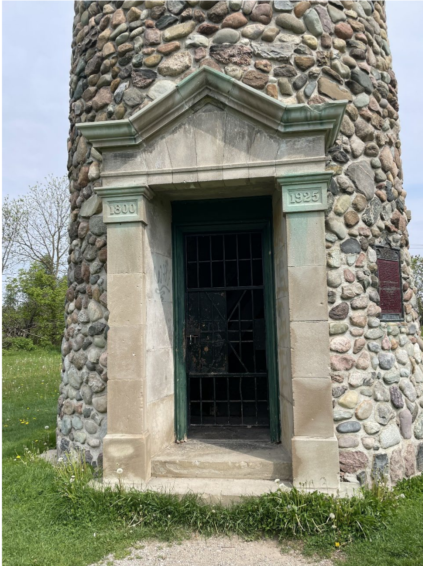
Figure 16: The base of the Waterloo Pioneer Memorial Tower, showing the limestone entrance and fieldstone veneer (A.S.I., 2024).
