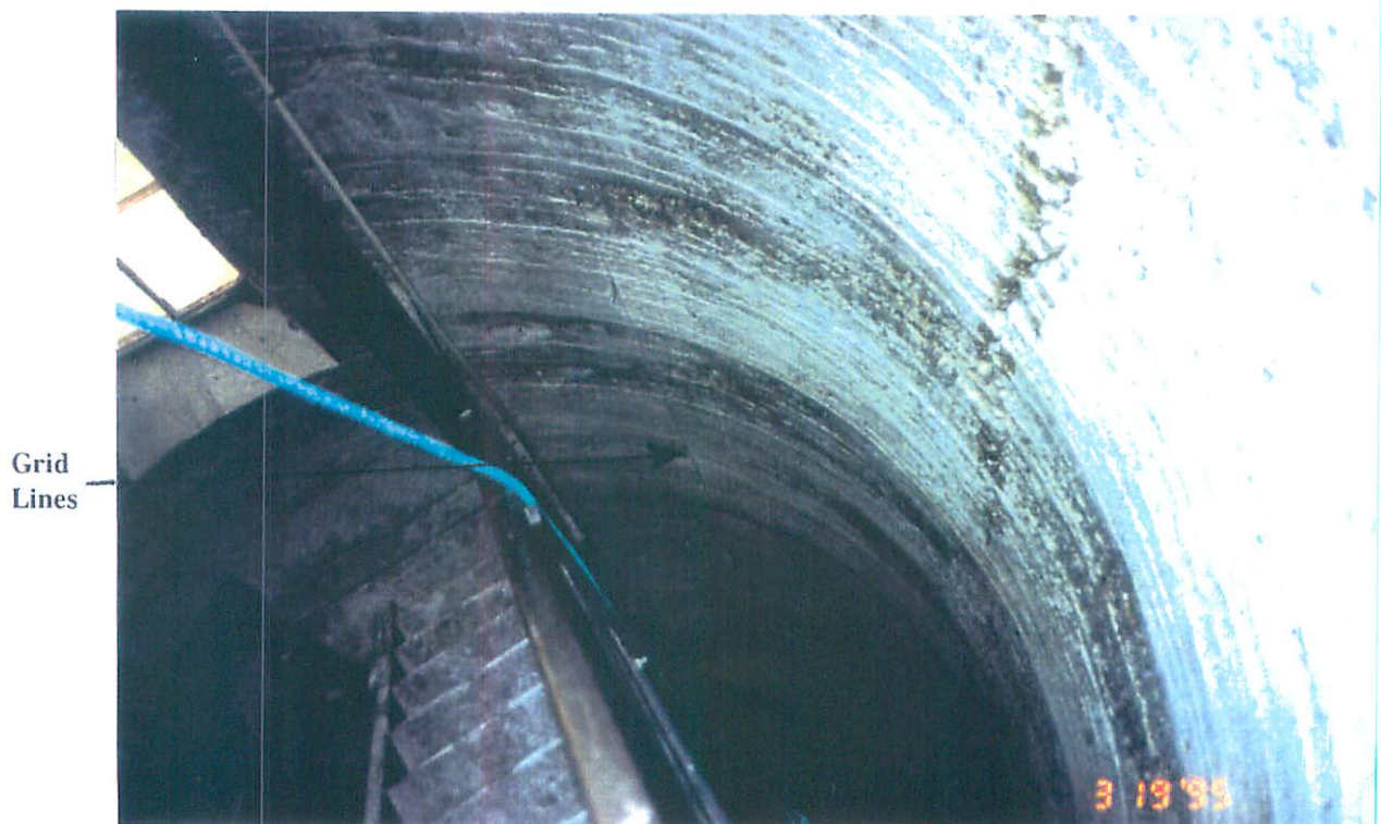
View of inside concrete surface from top of staircase (opposite entrance) Note: grid string lines
