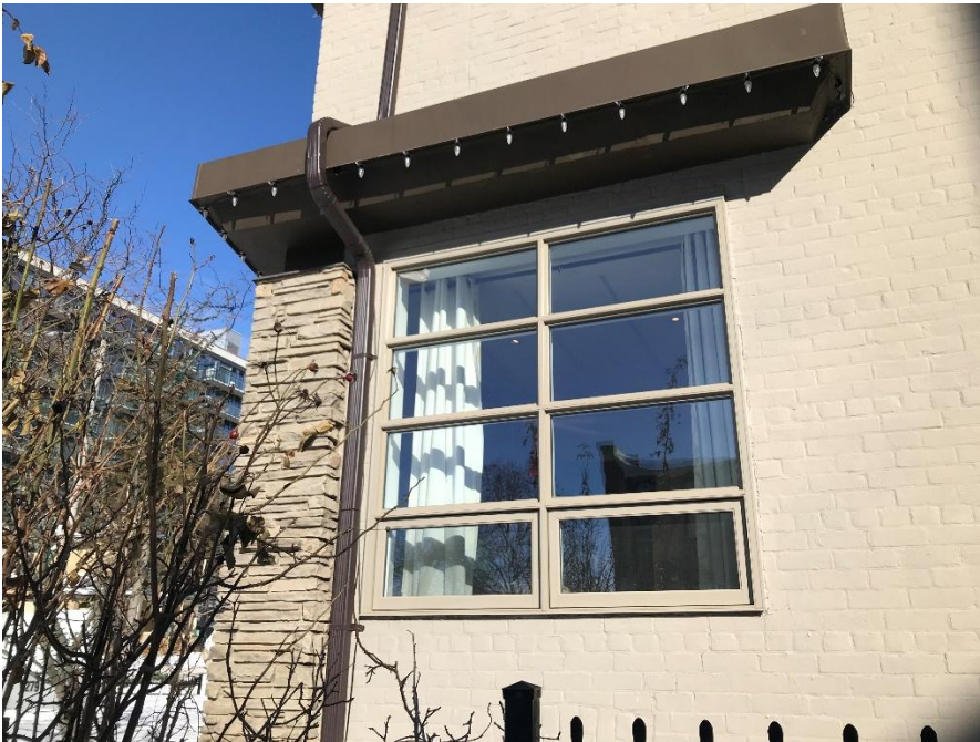
Detail of south (side) elevation showing lower window to be replaced with a replica of the original painted wood window.
