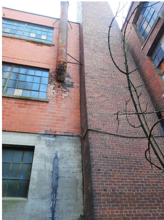
Photograph No. 9 –Chimney to Be Demolished and Brick Salvaged for Reuse
