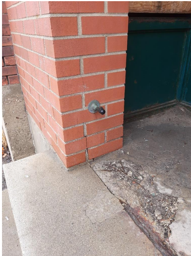
Photograph No. 2 – Right Entrance Floor Slab Deterioration
