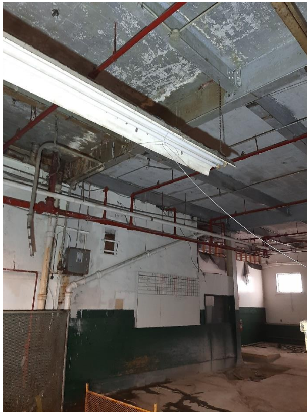
Photograph No. 41 – Ground Floor - Rain water leaking thru Concrete floor slab above
