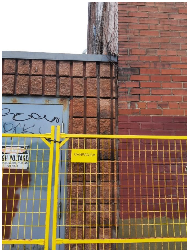
Photograph No. 4 – Brick Mortar Deterioration
