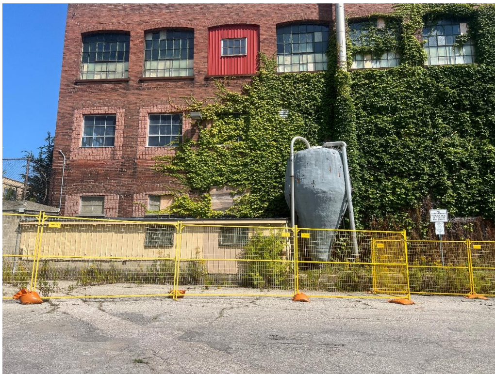
Photograph No. 7 – Overview of Non-matching Split Face Architectural Block and Red Sheet Metal Cladding Window Infills
