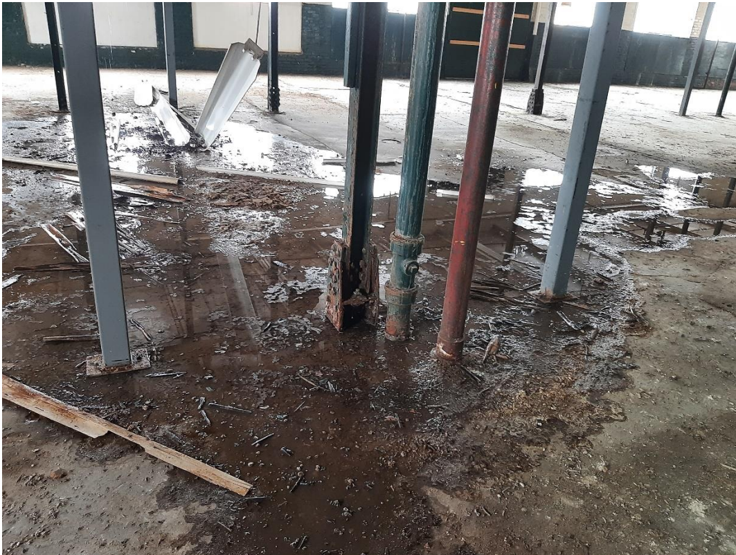
Photograph No. 53 – Third Floor - shoring in place since 2012
