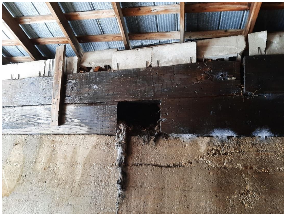
Photograph No. 62 – Courtyard, Timbers leaning, CMU Block at top
