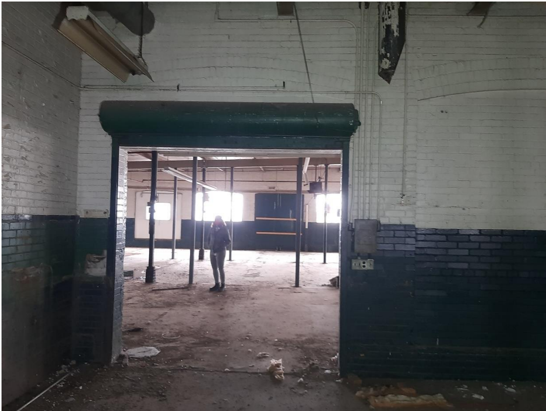
Photograph No. 29 – Third Floor Opening to be infilled
