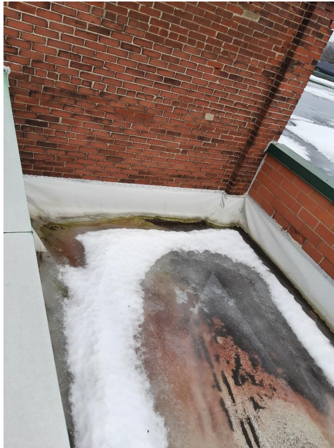
Photograph No. 34– Small roof over entrance stair, poor drainage
