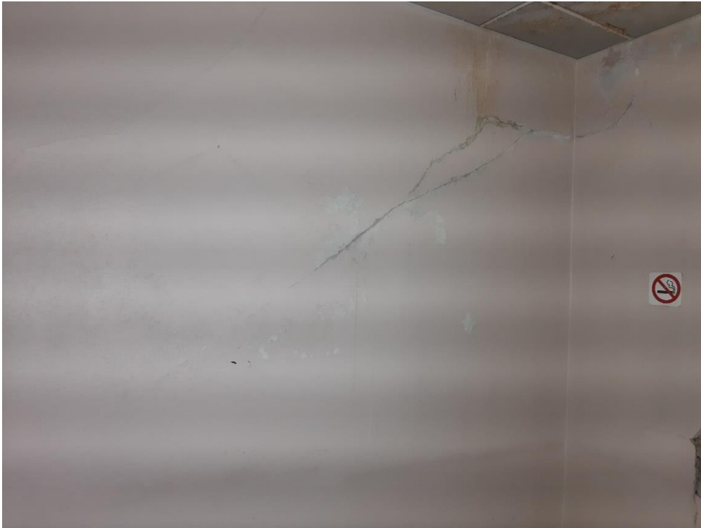
Photograph No. 50 – Second Floor - cracks in wall plaster
