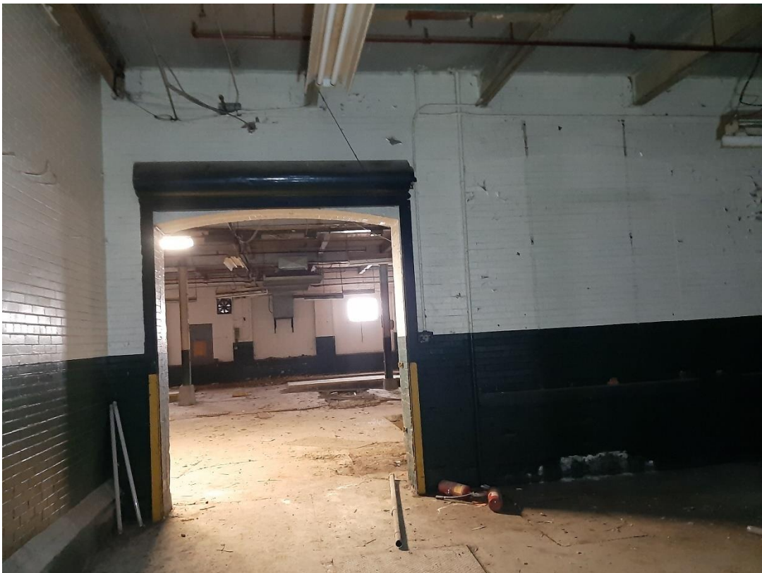
Photograph No. 14 – Ground Floor Door to be infilled
