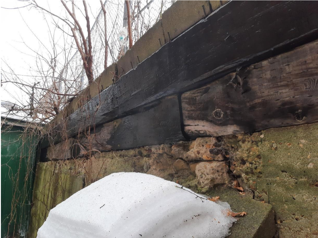
Photograph No. 65 – Courtyard, Timbers leaning, concrete deterioration
