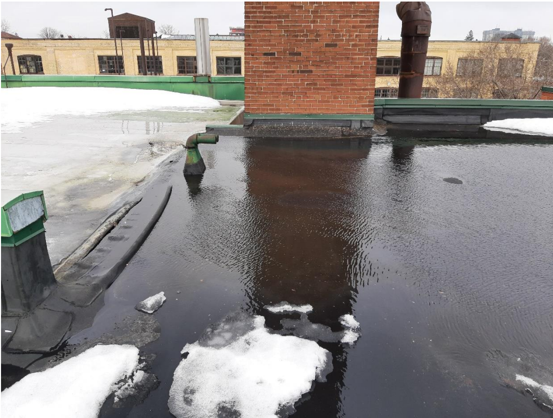
Photograph No. 38 – Edge of 1913 east wall, source of roof leak
