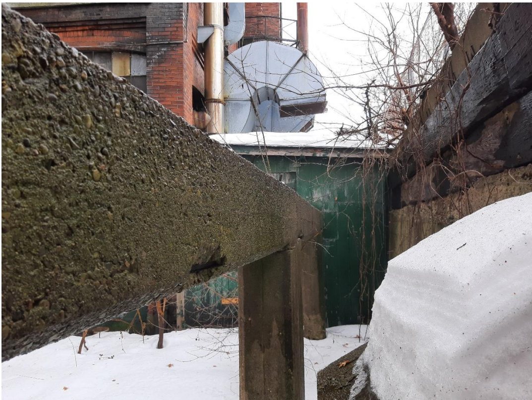
Photograph No. 66 – Courtyard, Timbers leaning, rot
