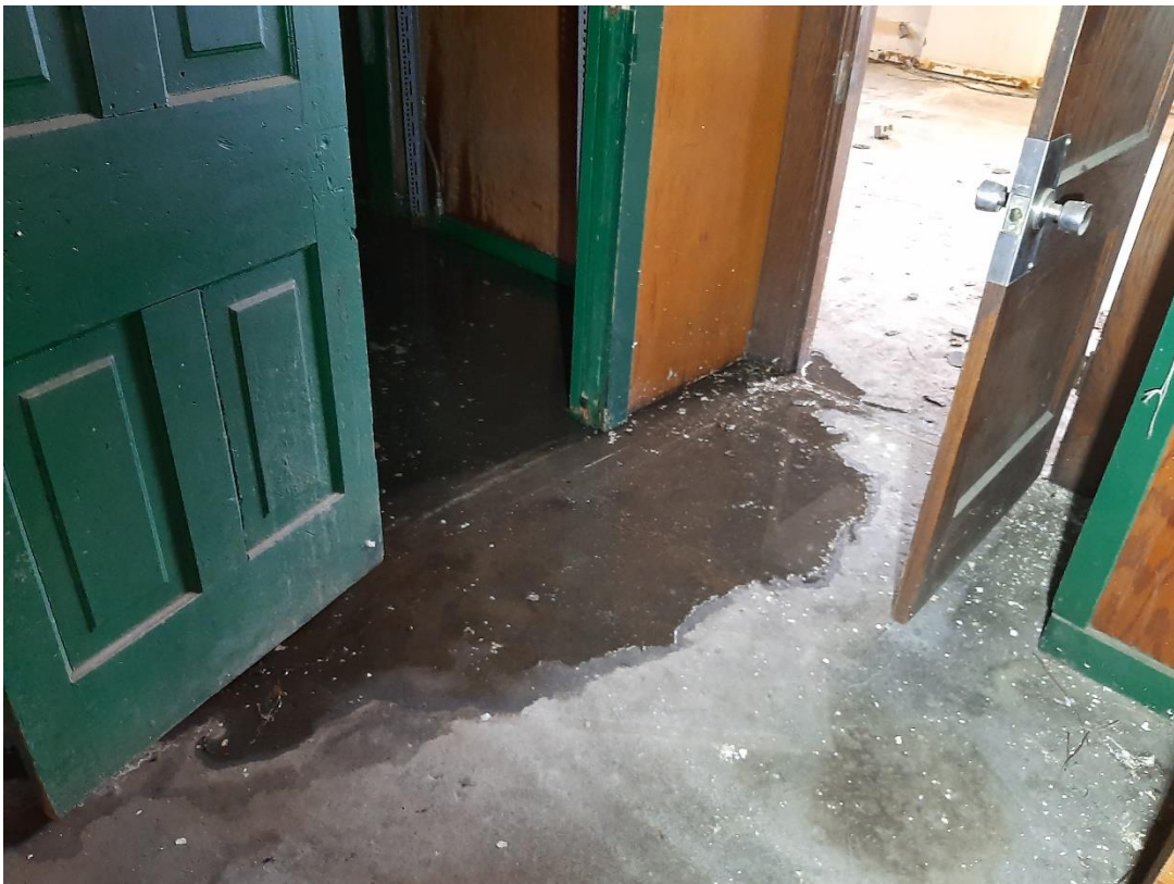
Photograph No. 48 – Second Floor, Water leak from roof
