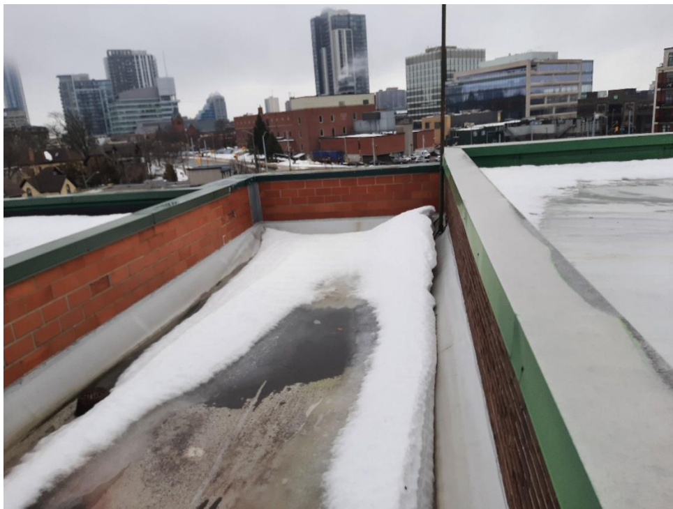
Photograph No. 35 – Small roof over entrance stair, poor drainage
