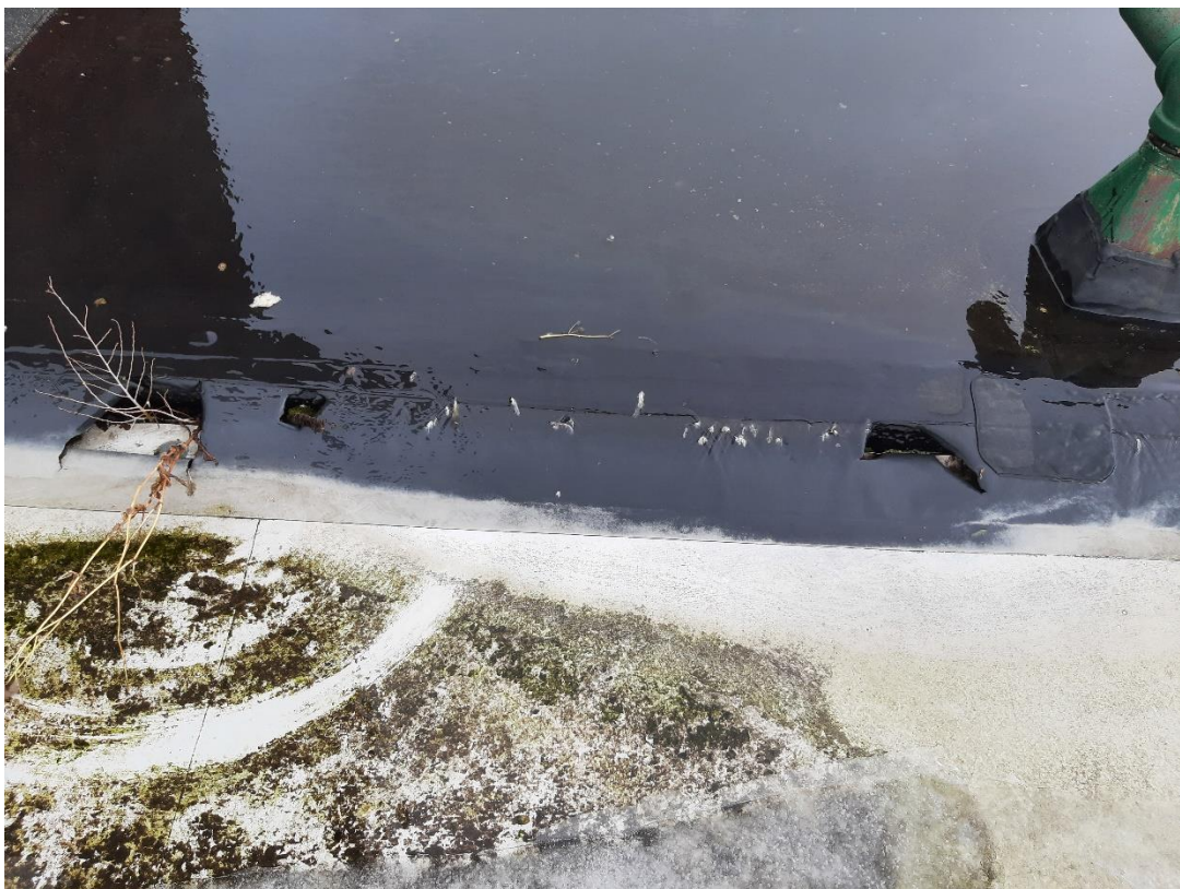
Photograph No. 37 – Edge of 1913 east wall, source of roof leak
