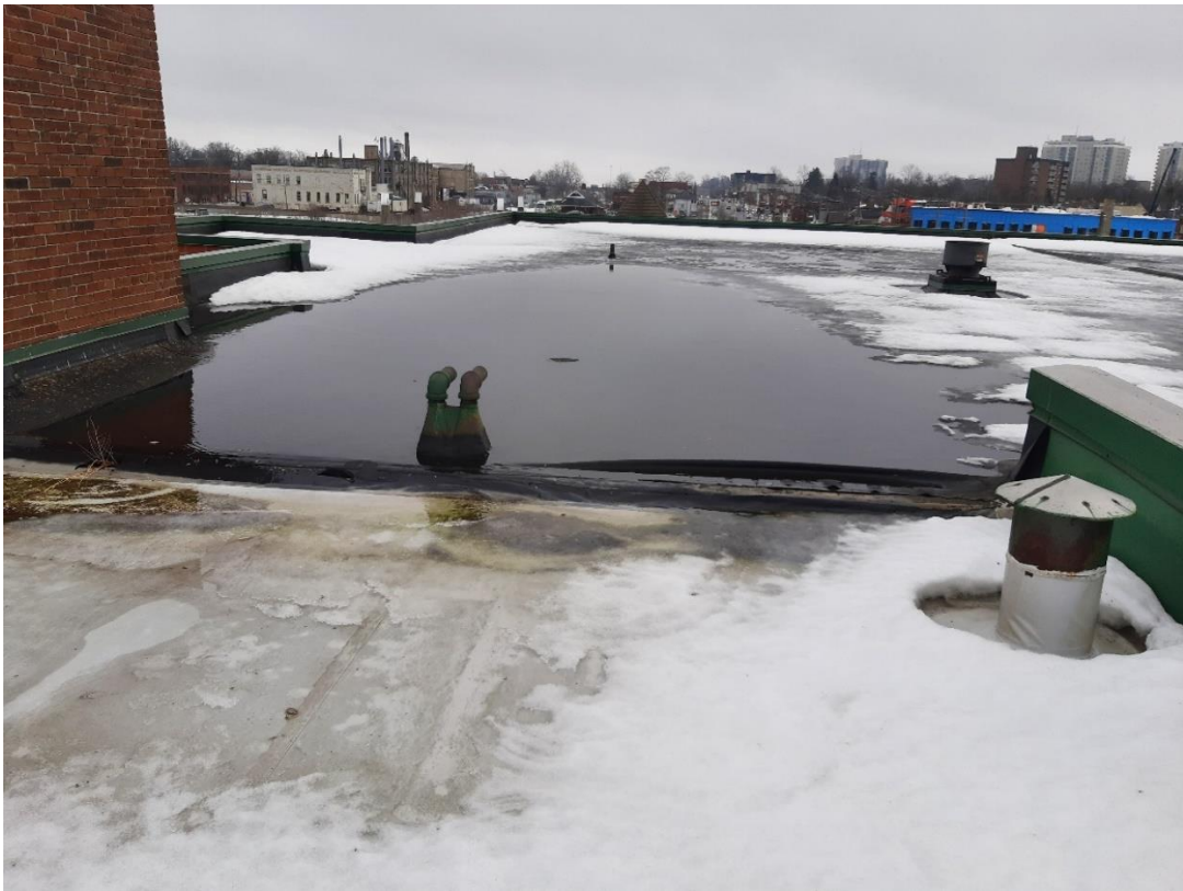
Photograph No. 36 – Edge of 1913 east wall, source of leak
