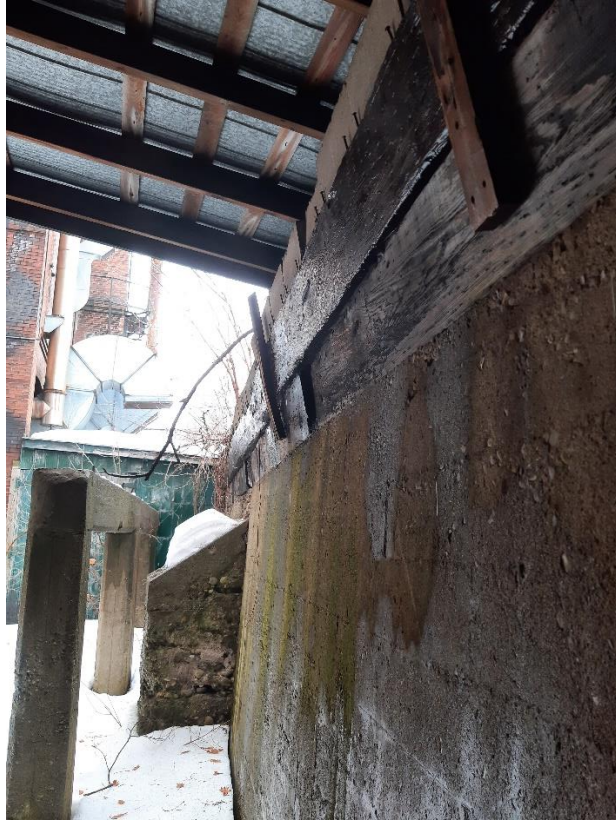
Photograph No. 63 – Courtyard Wall, Looking west, Timbers leaning, Vulnerable CMU Block at top
