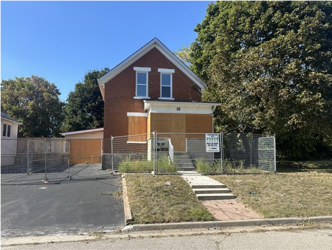
Figure 4: View of the Existing Duplex at 16 Reinhardt Street
