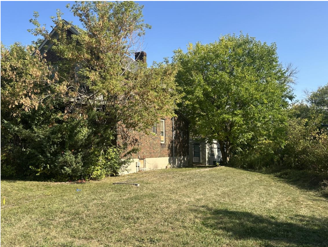
Figure 3: Side View of the Existing Dwelling at 15 Reinhardt Street
