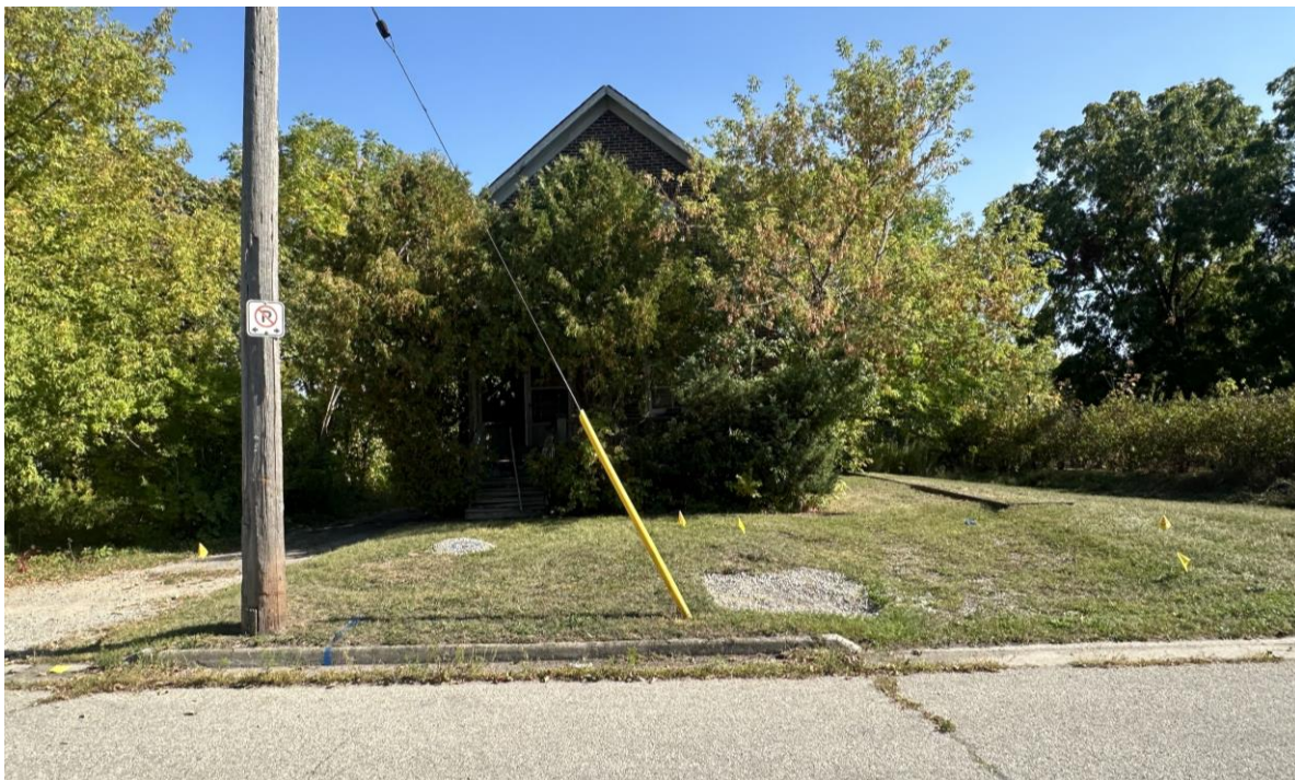
Figure 2: Front View of the Existing Dwelling at 15 Reinhardt Street
