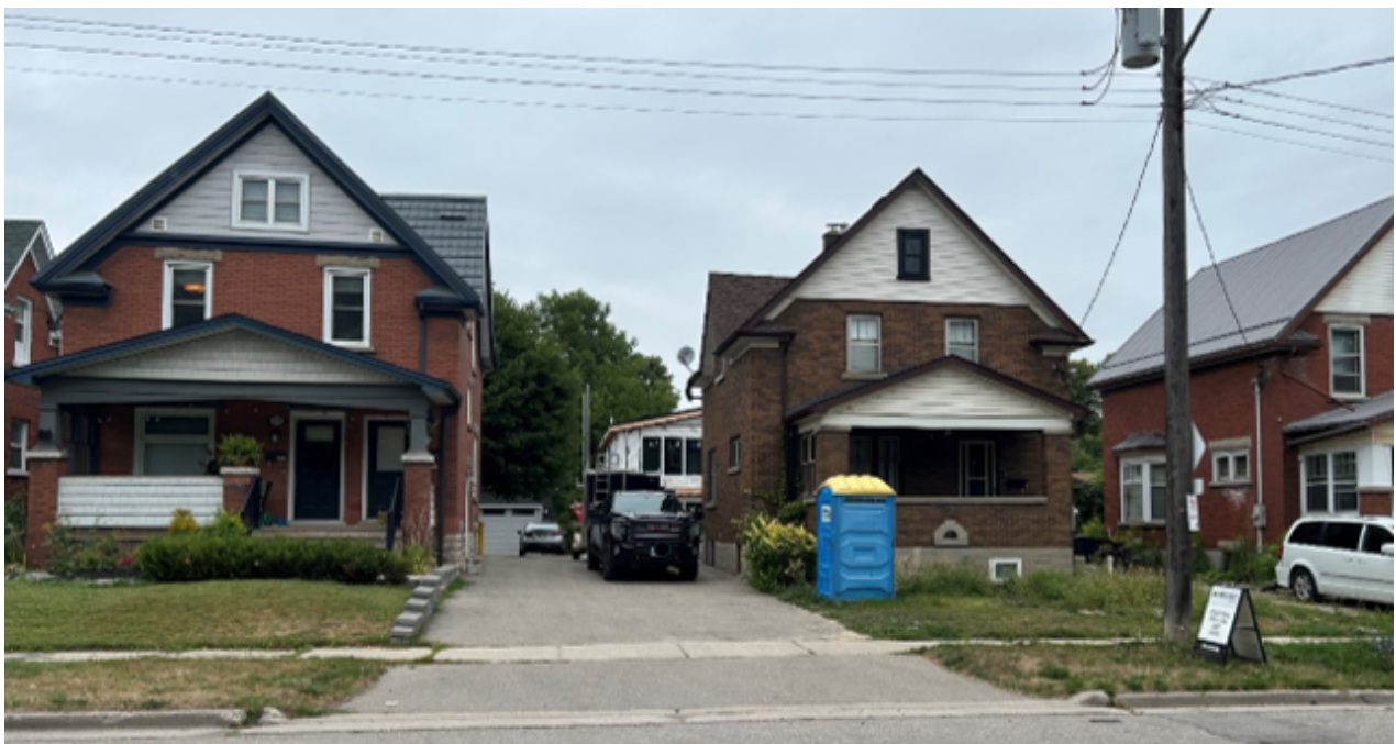
356 Wellington Street North - Duplexed principal dwelling and duplexed backyard home under construction (4 units total)
