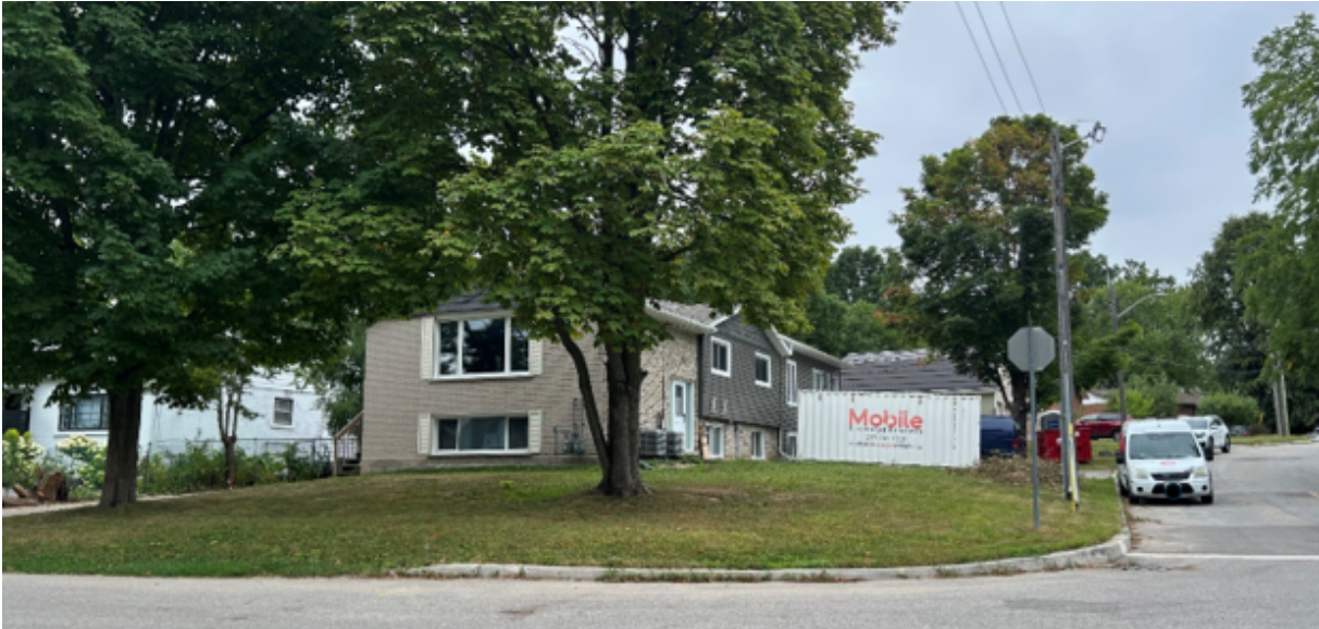
1 Horizon Court – fourplex in renovated single detached dwelling
