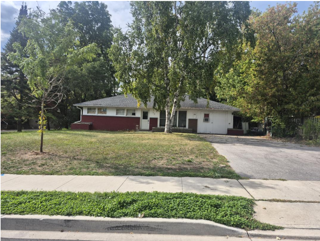
Existing building at 32 Windom Road
