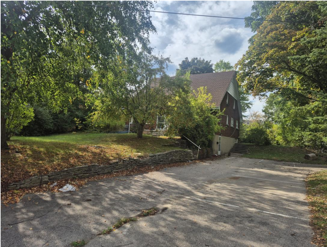
Existing building at 42 Windom Road
