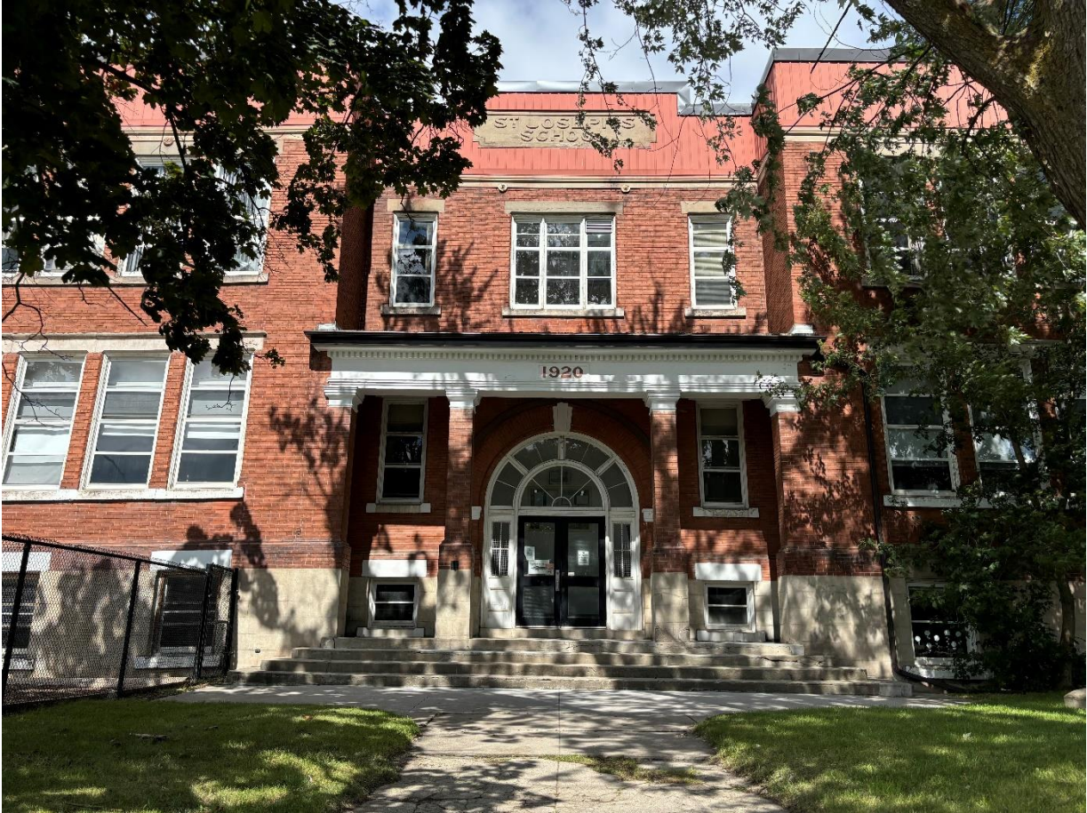
Figure 2. Front Façade of the School.
