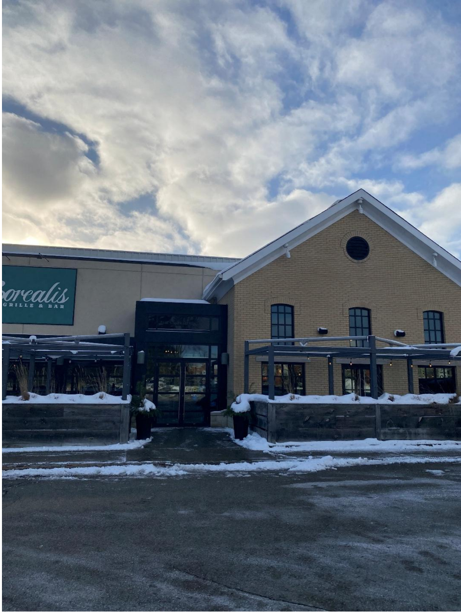
4336 King Street East: Rear Addition Facade
