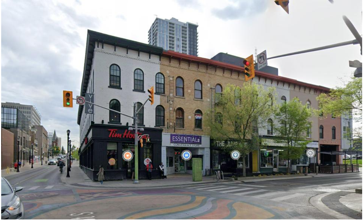
Front Façade of 8-24 King Street East.
