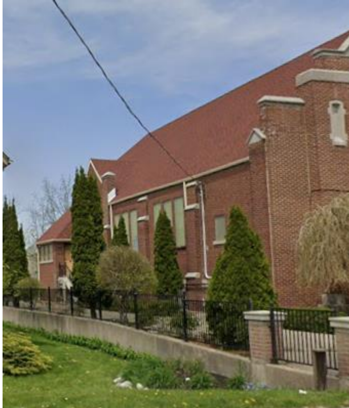
Side Elevation (South Façade) (Google, May 2025)
