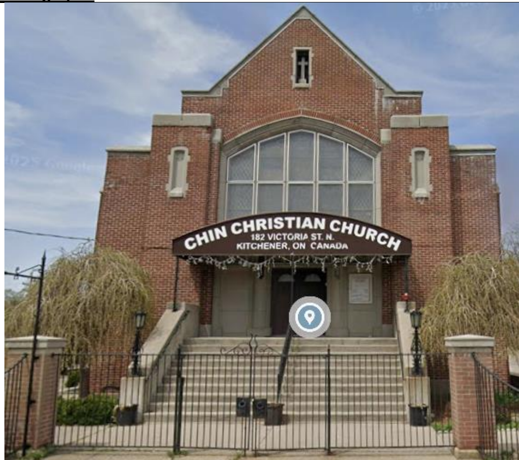
Front (Victoria Street North) Elevation (East Façade) (Google, May 2025)
