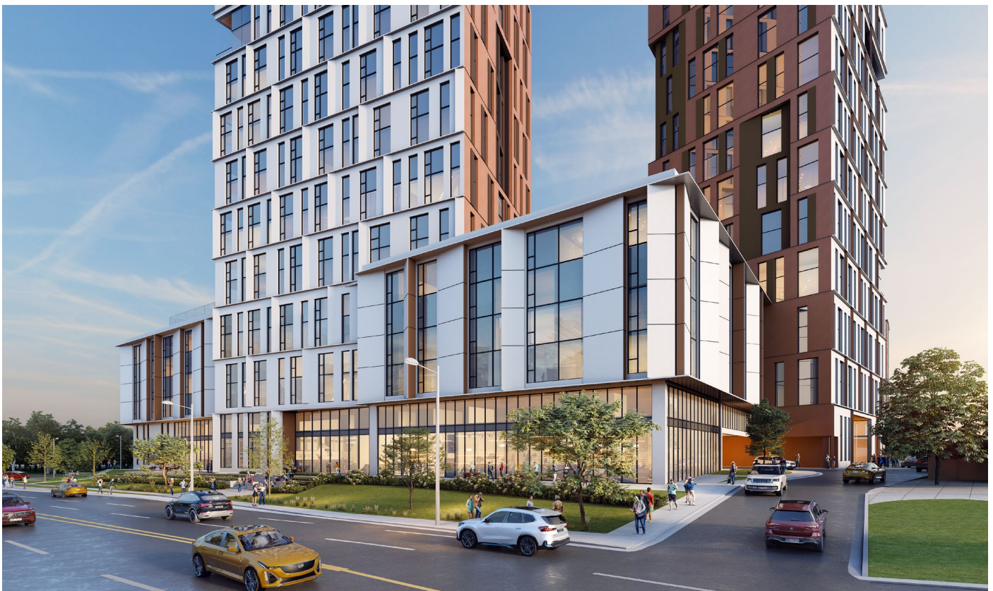
FIGURE: Rendering showing the active and transparent podium base's face along the Courtland Avenue East frontage (ABA Architects).
