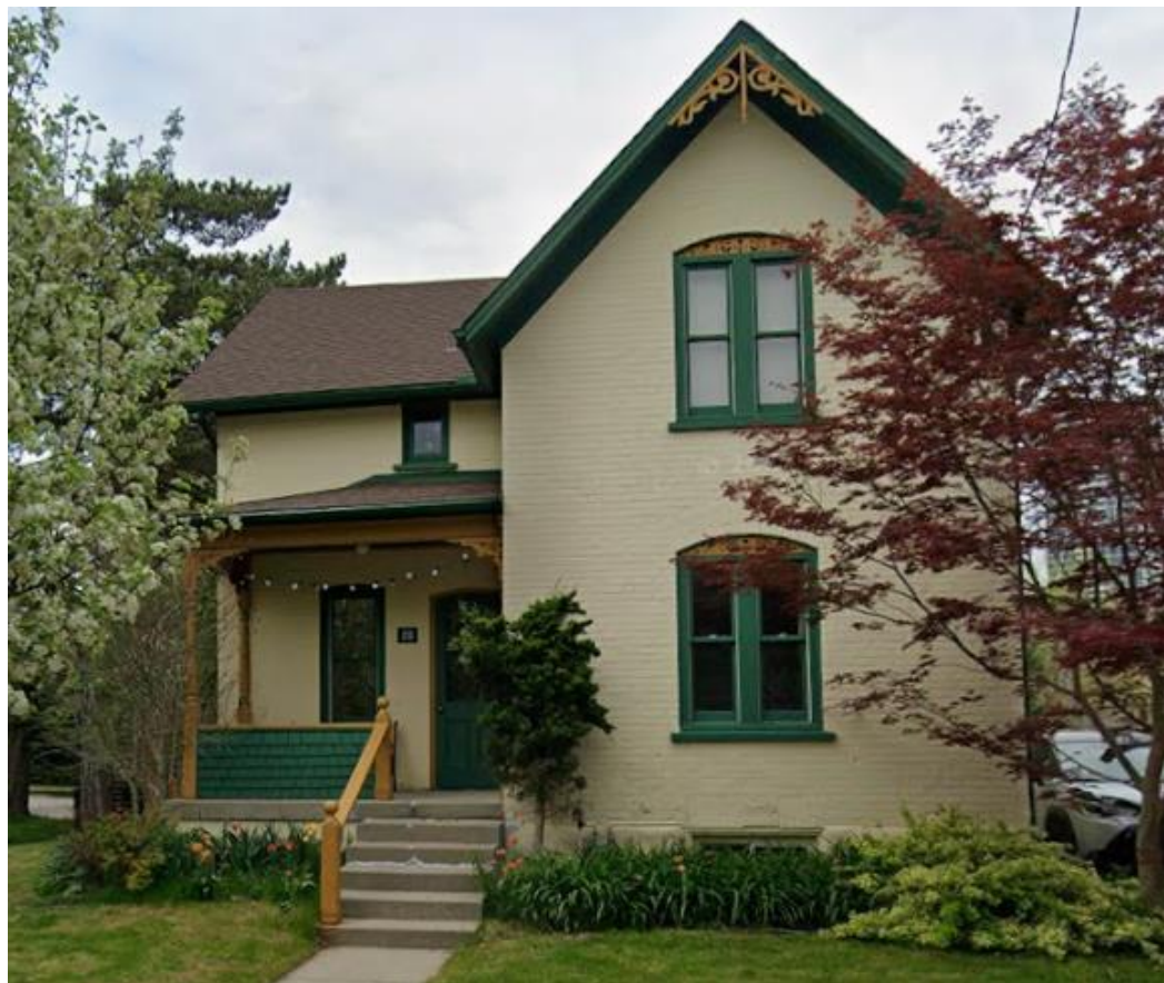
Front (Linden Avenue) Elevation (Southeast Façade)
