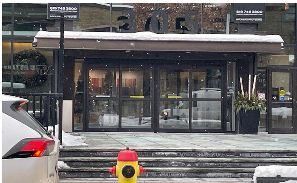
Front Entrance (North Façade) – 305 King Street West
