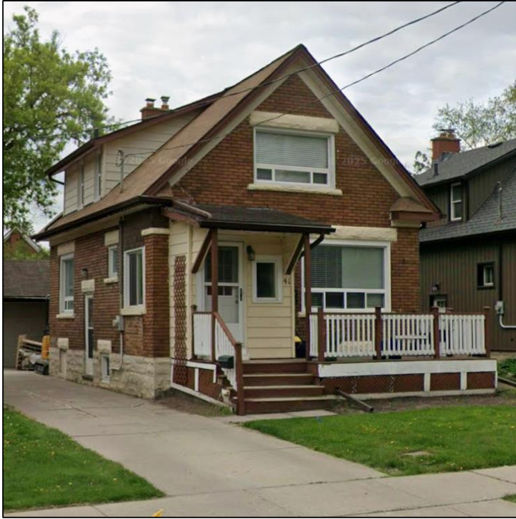
Figure 2: Front Façade of 41 Michael Street
