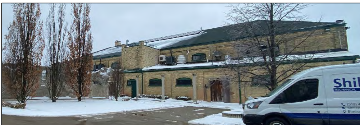
Figure 27: Image of east elevation of Building 1 (MHBC, 2023).
