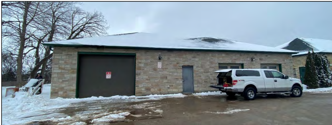
Figure 37: Image of west elevation of Building 3 (MHBC, 2023).
