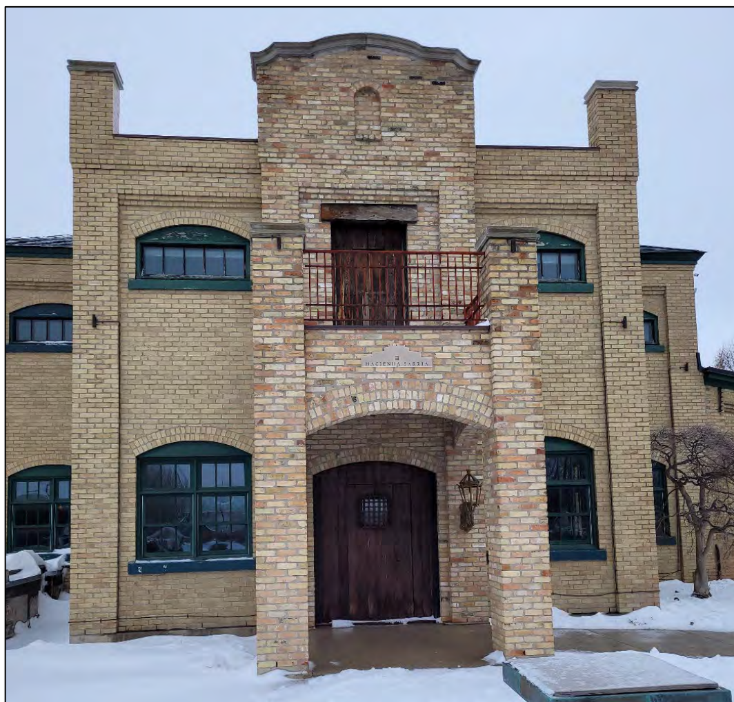
Figure 24: Image of additions on south elevation of Building 1 (MHBC, 2023).
