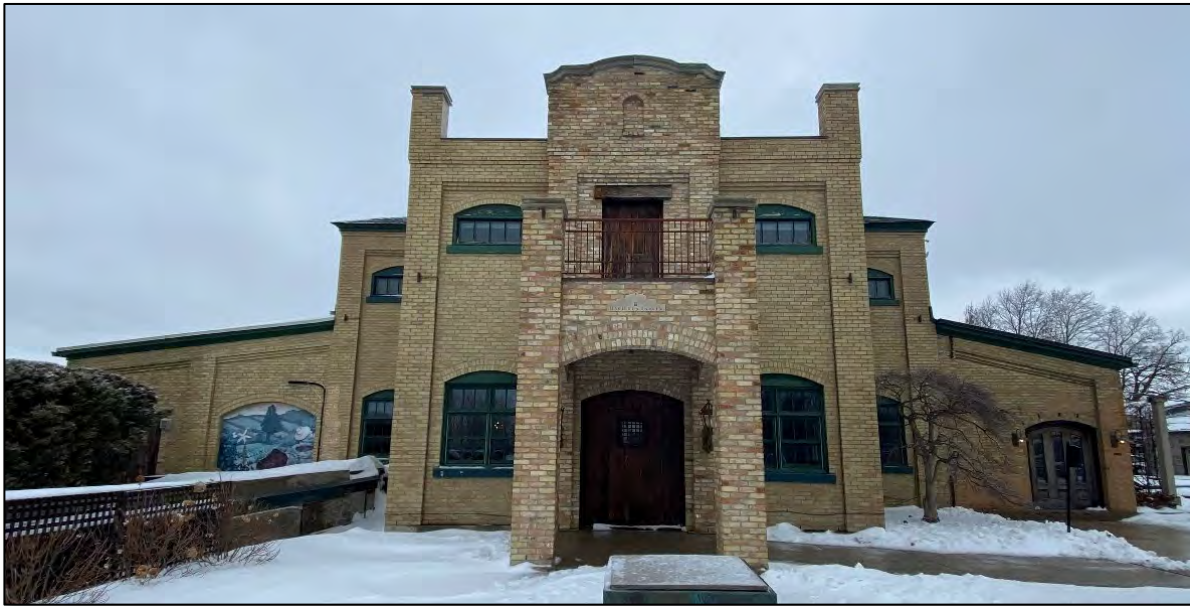
Figure 23: South elevation of warehouse building (Building 1) (MHBC, 2023).
