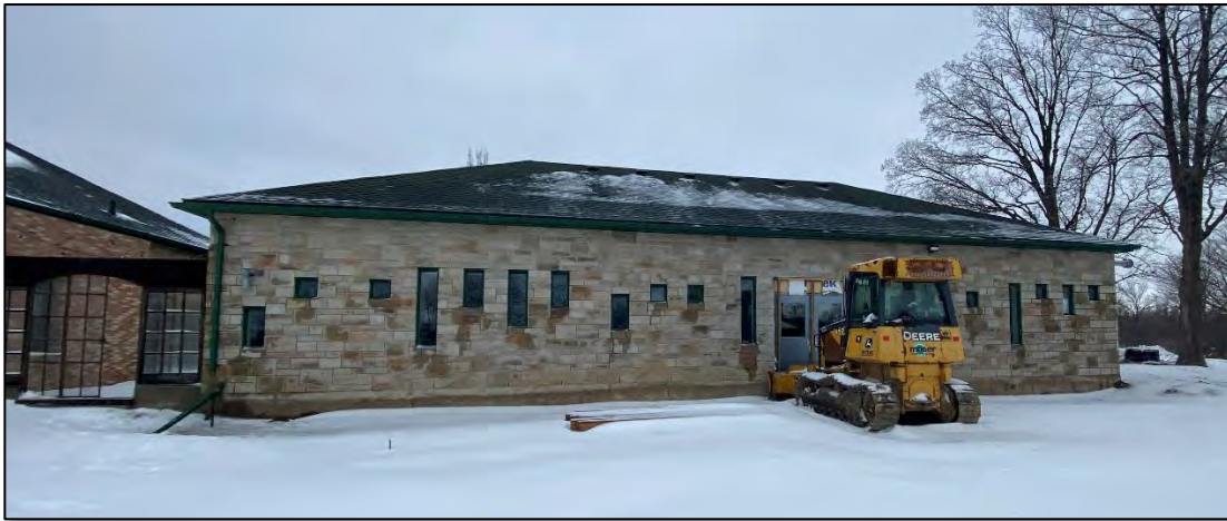
Figure 40: Image of west elevation of Building 3 (MHBC, 2023).
