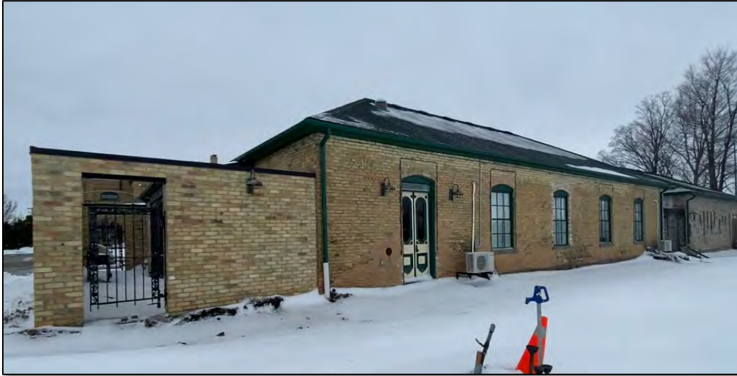
Figure 36: Image of east elevation of Building 2 (MHBC, 2023).
