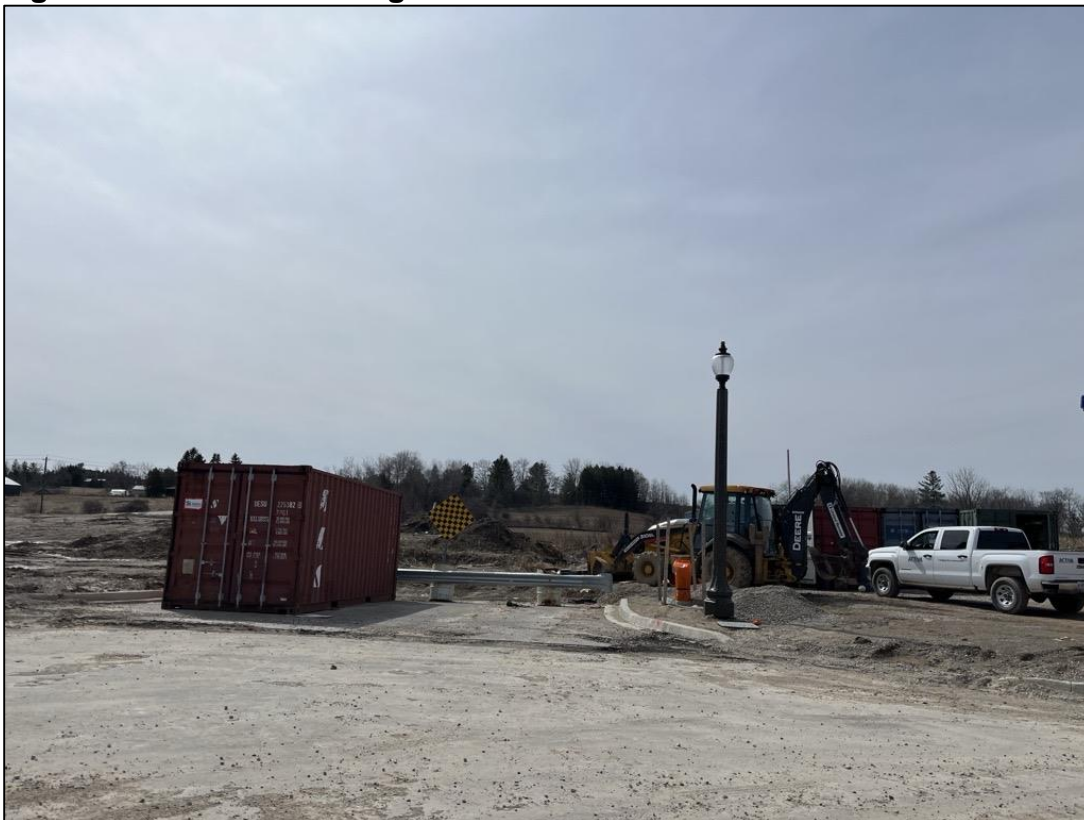
Figure 3 – View of Existing Site
