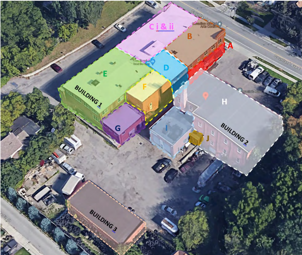
Figure 30: Aerial photo of the subject property identifying the location of sections of Buildings 1, 2, and 3. (Source: Google Earth Pro, accessed 2024)
