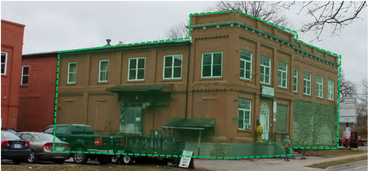
Figure 48: View of Building 1 (east and north elevations) noting portion proposed for retention and conservation (Source: MHBC, 2024)
