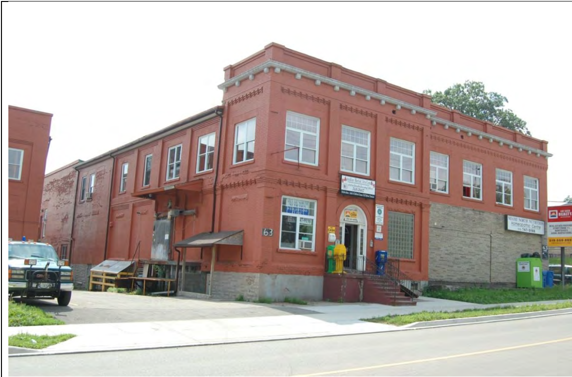
63 Courtland Avenue East – Front Elevation
