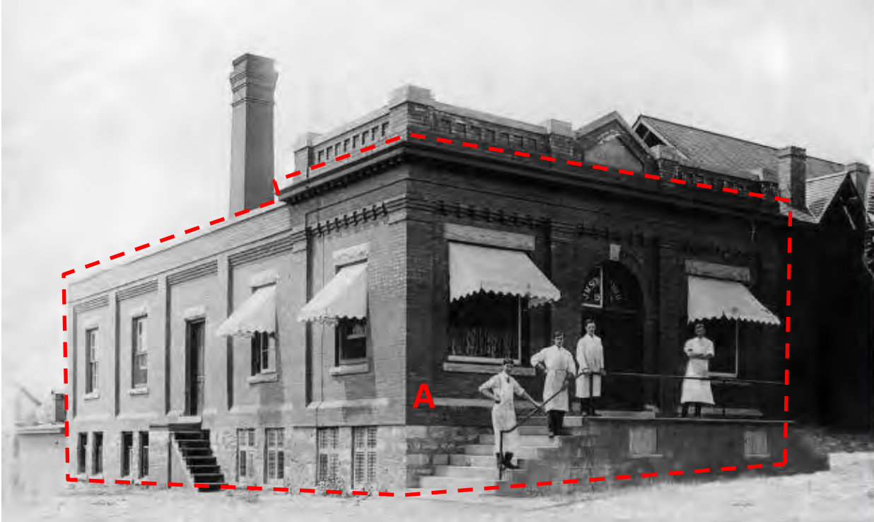
Figure 13: Photograph of the J.M. Schneider factory addition (“Meat Market”) formerly located on the subject property, c. 1909. This portion of the building is identified in this report as Section “A” (Source: Kitchener Public Library)
