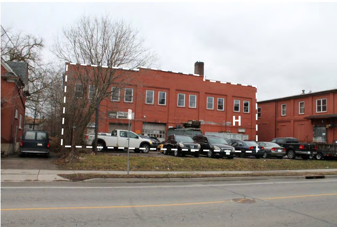
Figure 35: View of north (front) elevation of Building 2 fronting Courtland Street East (MHBC, 2024)
