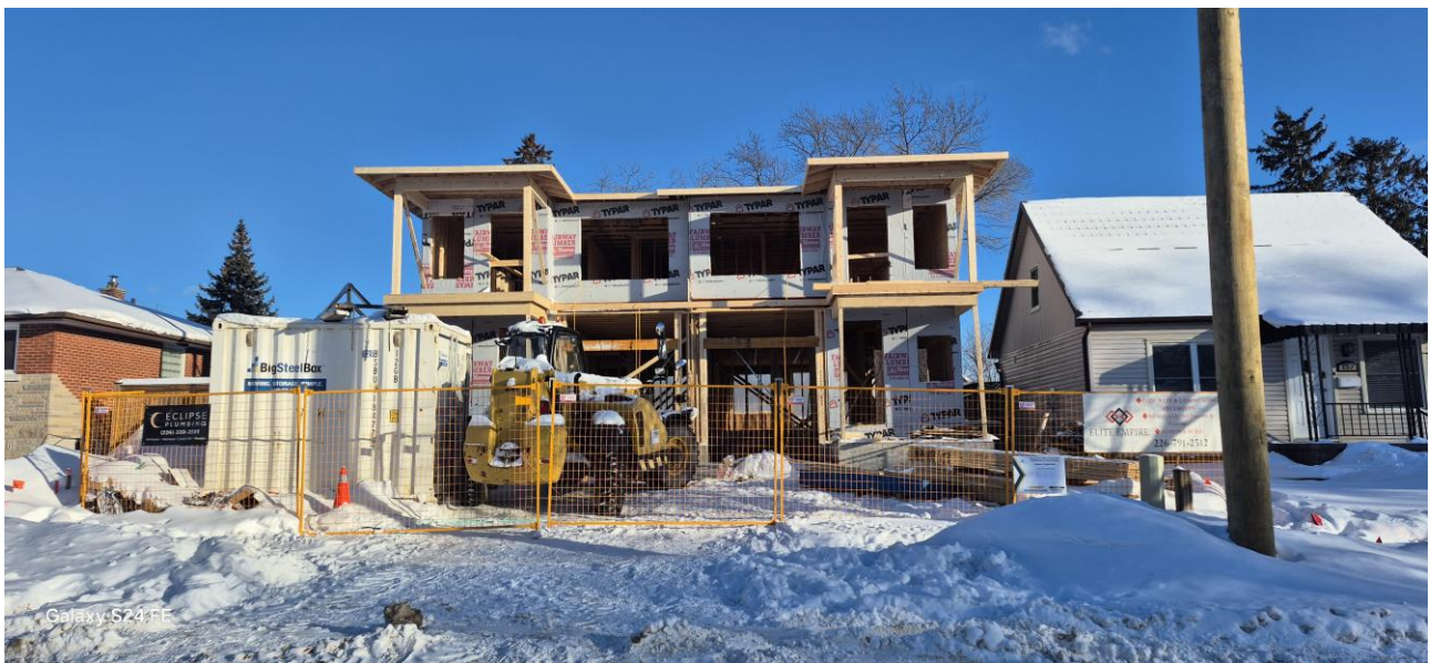
Figure 4: Photo of Front View of Semi-Detached Duplex Under Construction
