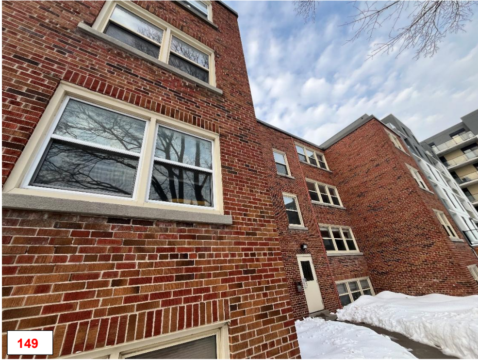
Rear Elevations (South Façade)
