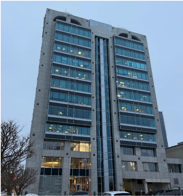
Rear Elevation (Halls Lane)
