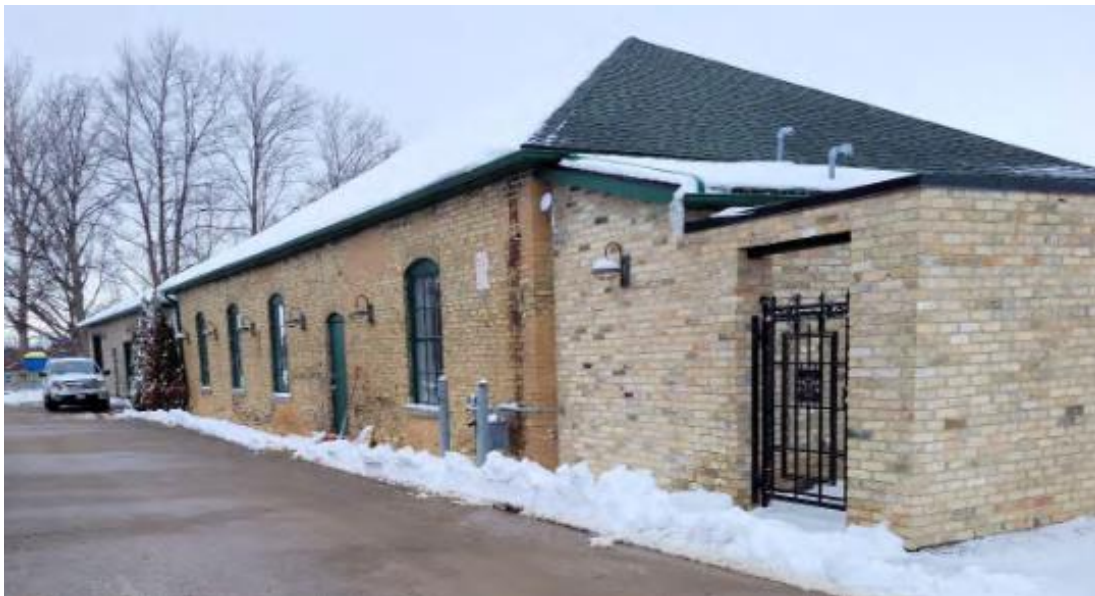
Figure 4. Former Machine Shop
