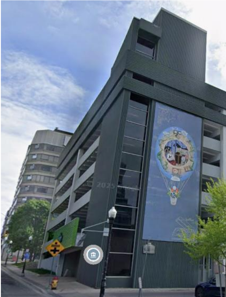
Halls Lane Elevation (South Façade) – 33 Ontario Street South (Google, May 2025)
