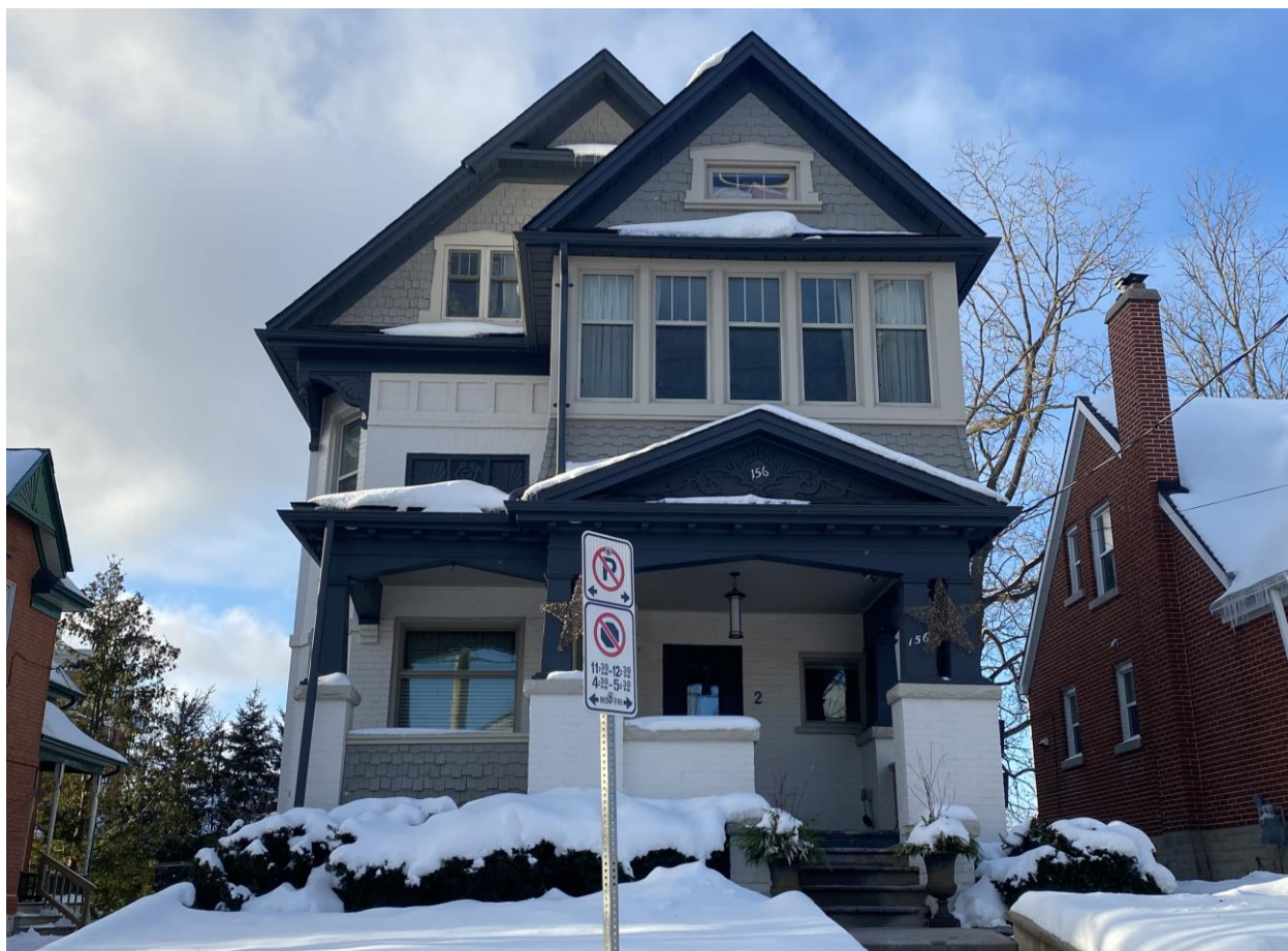
Figure 2.0: Front Elevation of 156 Benton Street
