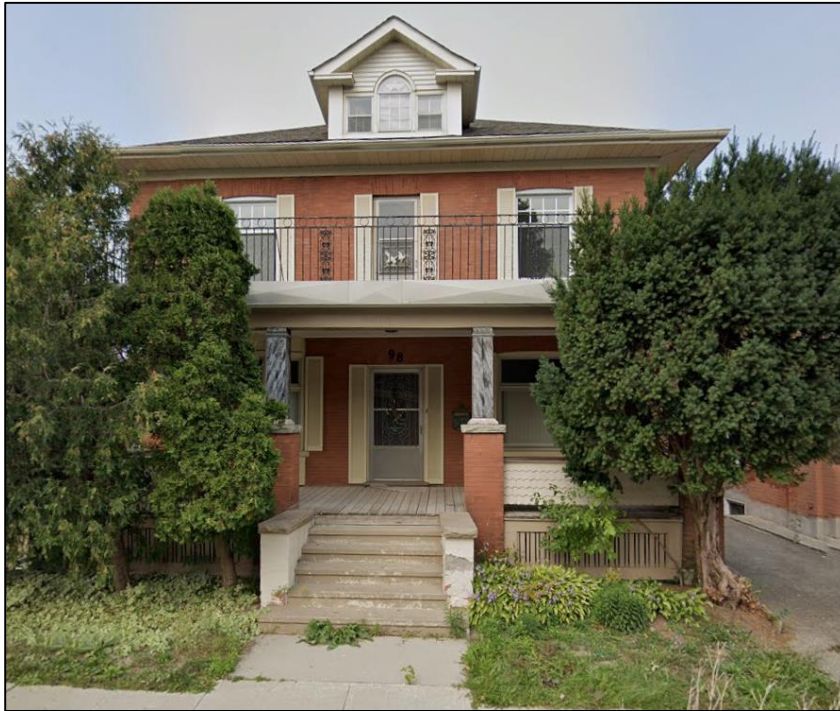
Figure 2: Front Façade of 98 College Street
