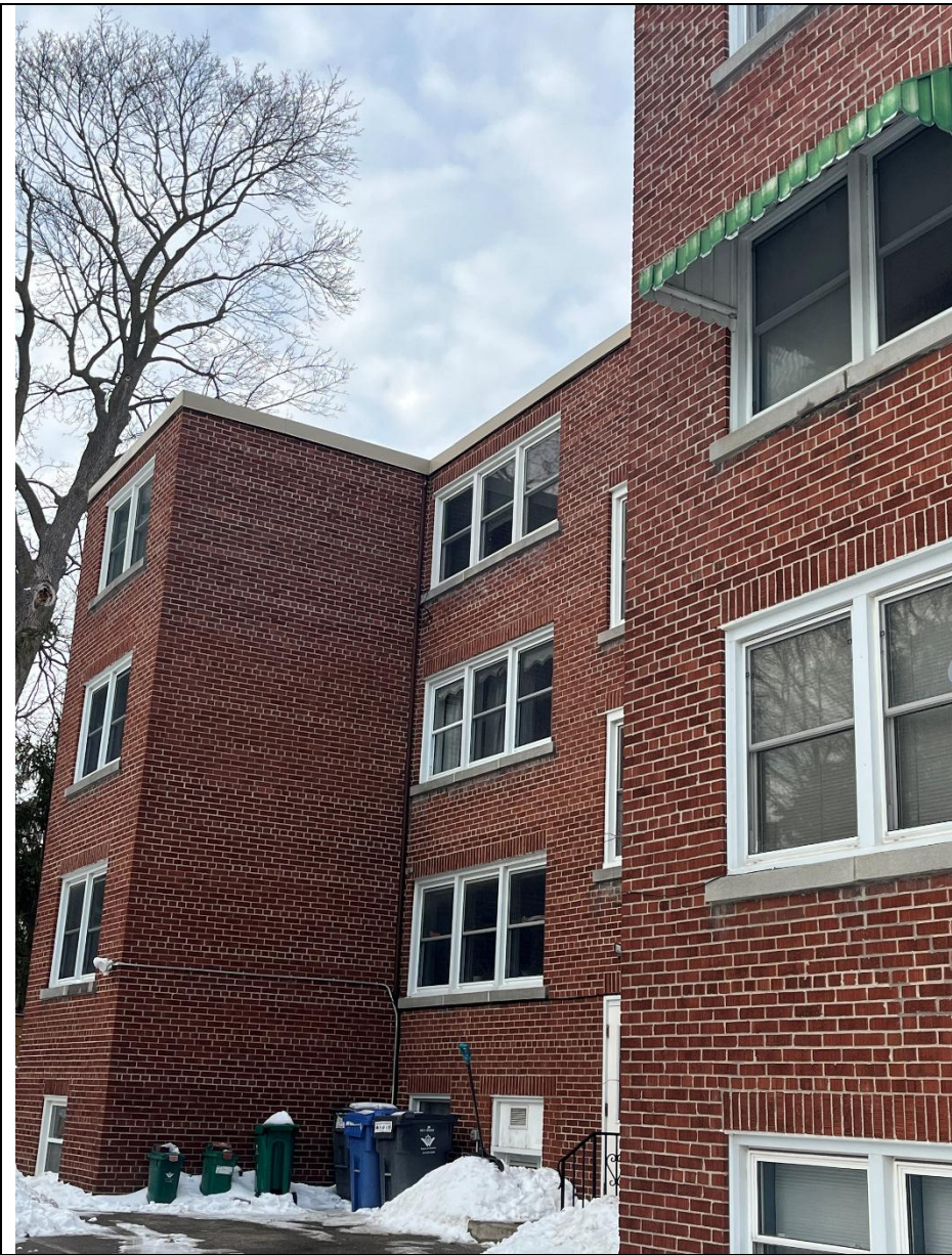
Rear Elevation (South Façade)
