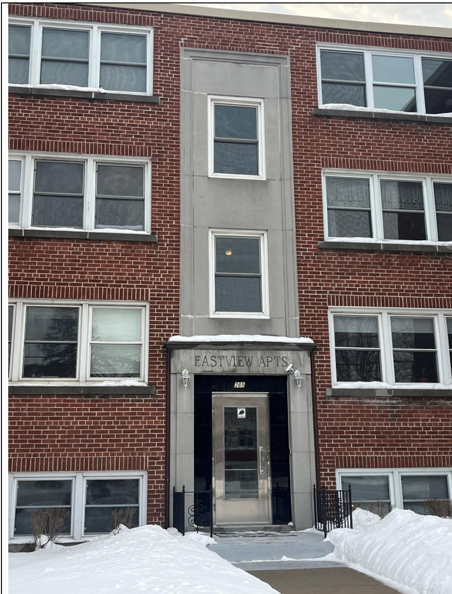
Detailing of front entrance portal
