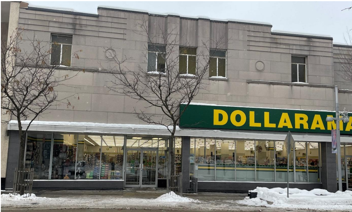
Front Elevation (North Façade) – 53-61 King Street East
