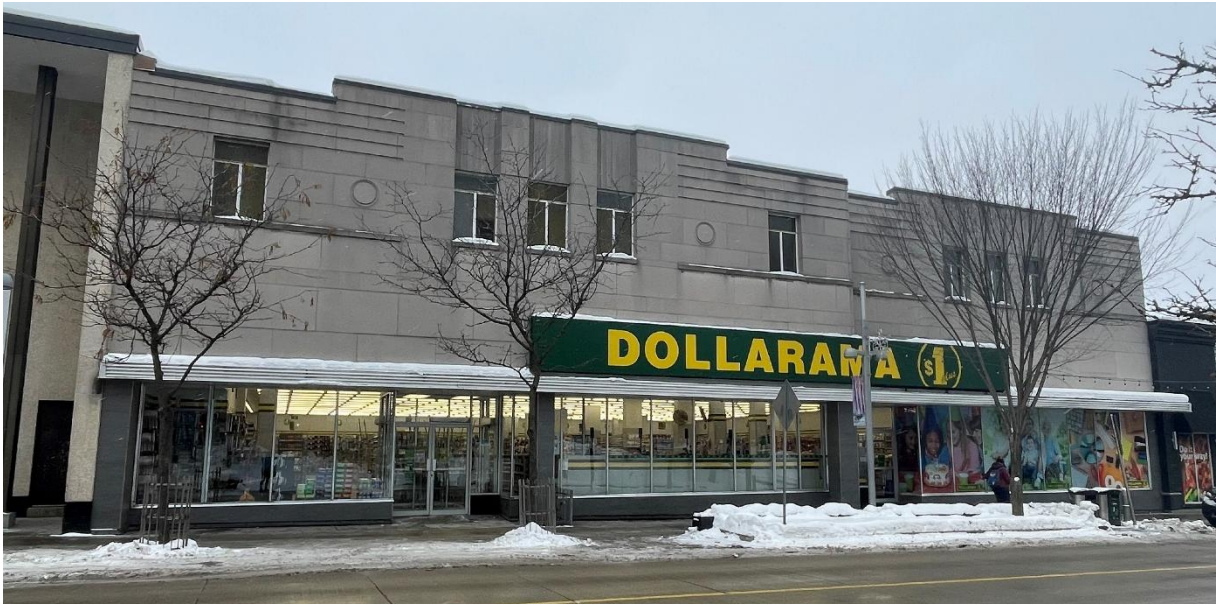
Front Elevation (North Façade) – 53-61 King Street East
