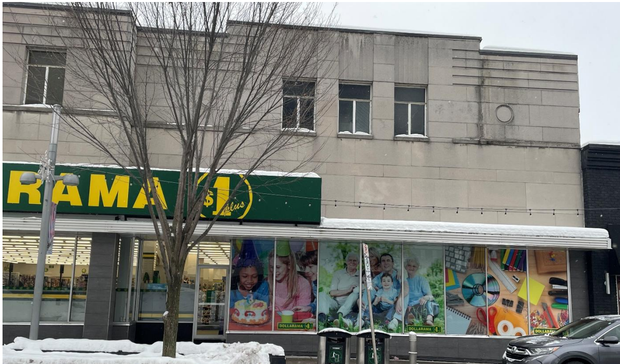
Front Elevation (North Façade) – 53-61 King Street East
