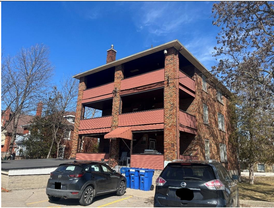
Rear Elevation (East Façade)
