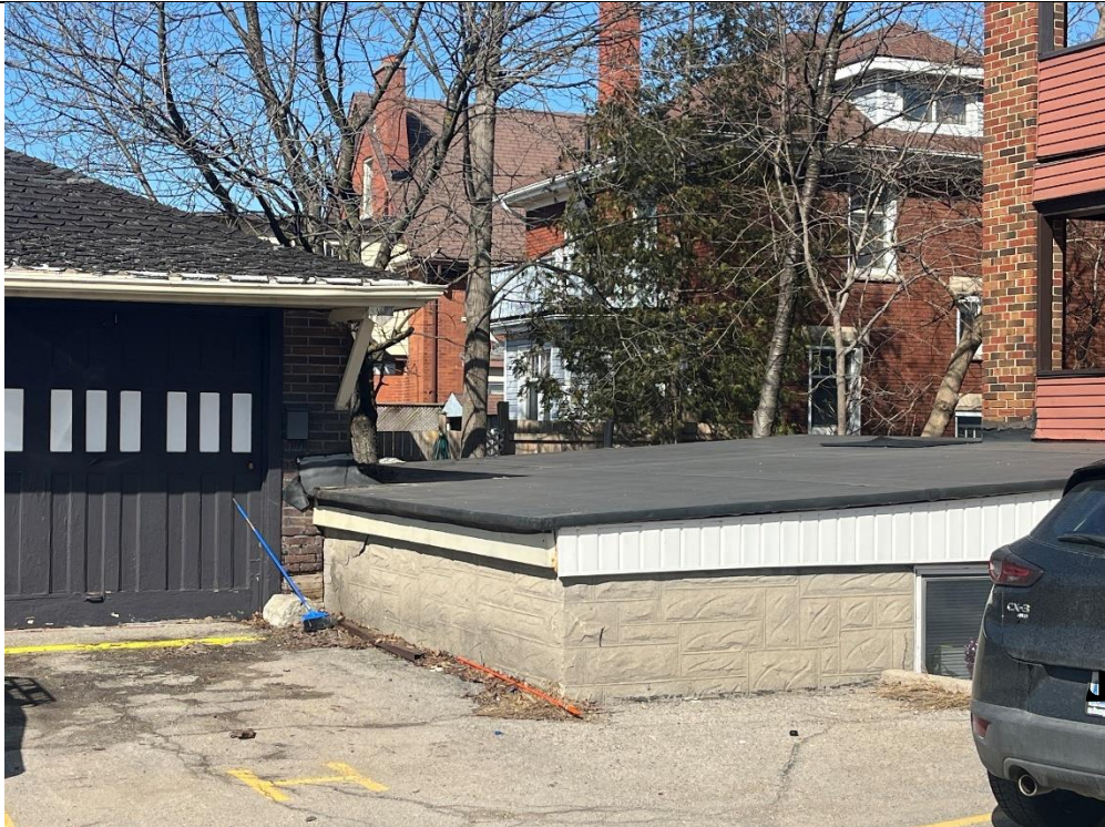
Detailing of covered basement
