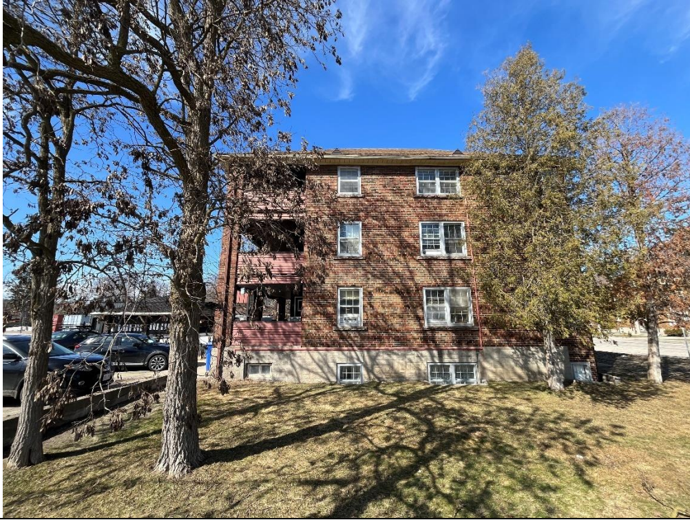
Side Elevation (North Façade)
