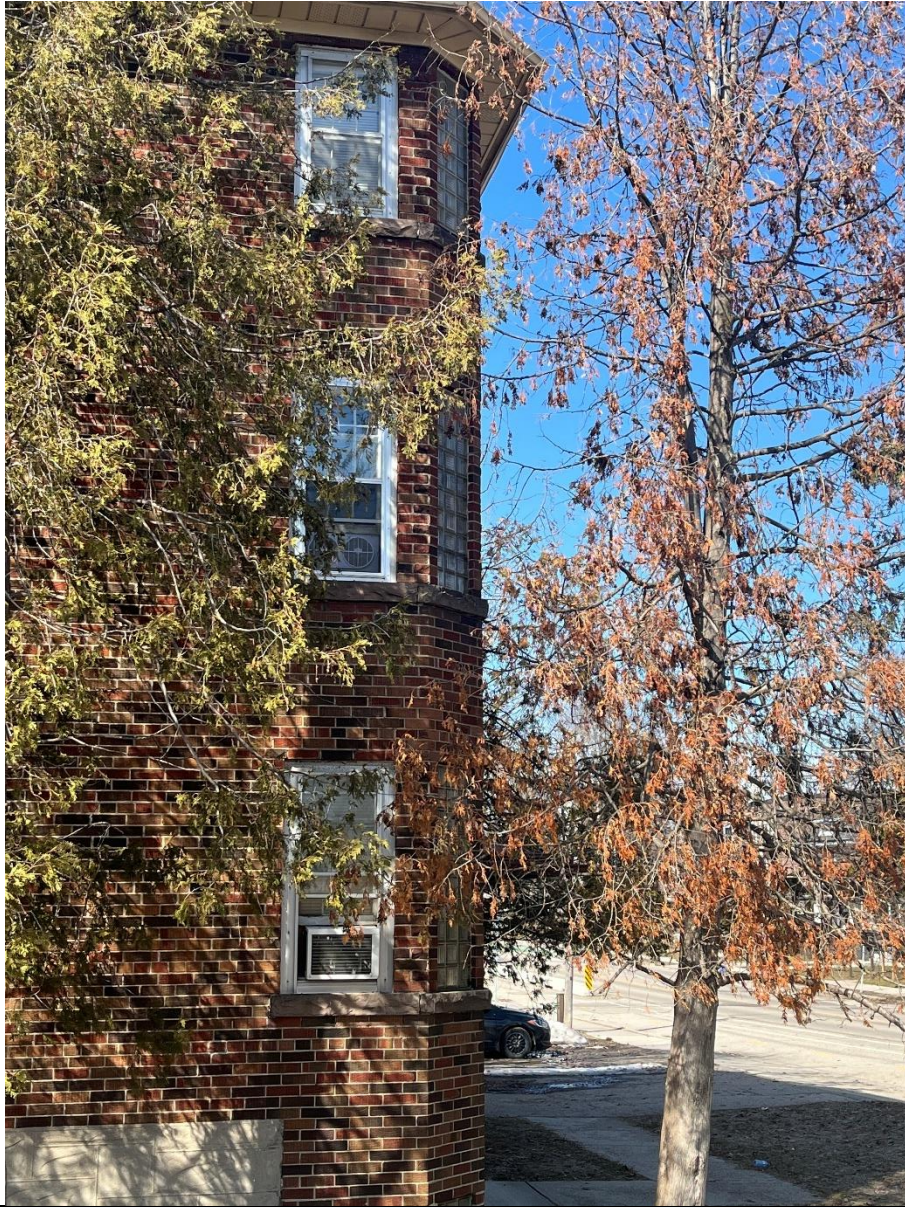
Detailing of angled corner with glass block windows
