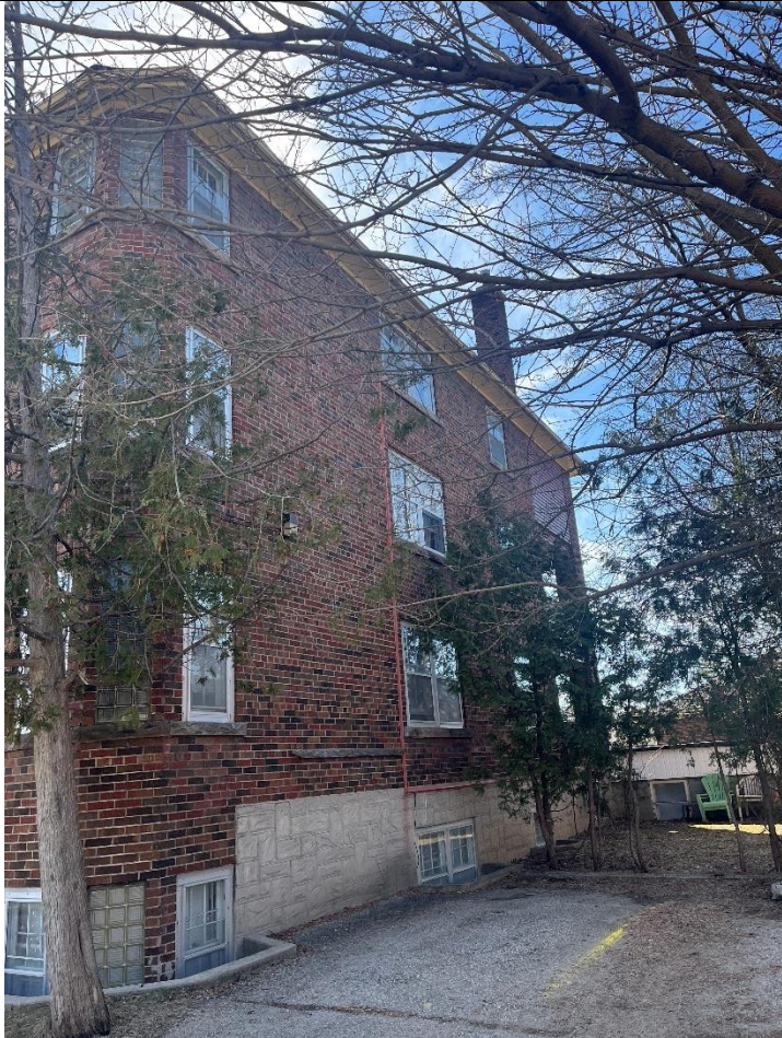
Side Elevation (South Façade)
