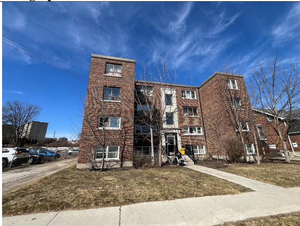
Front Elevation (South Façade)
