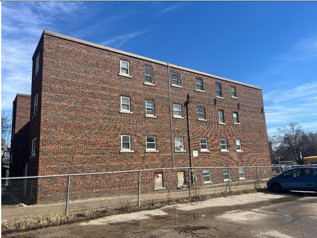
Side Elevation (West Façade)
