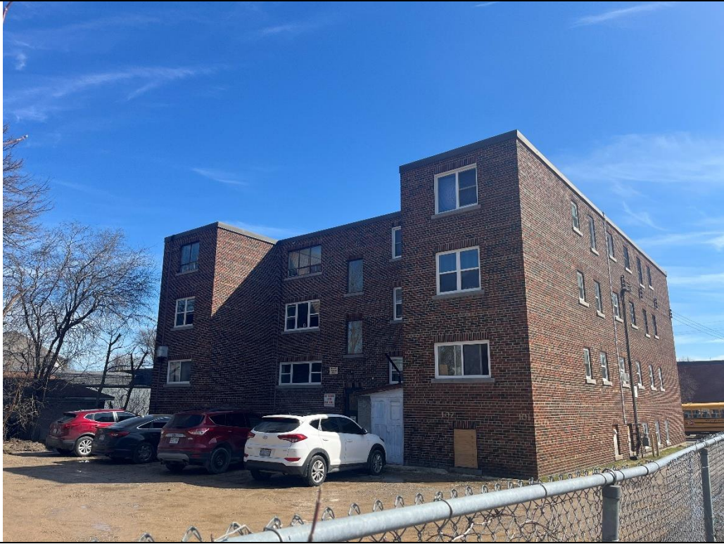
Rear Elevation (North Façade)
