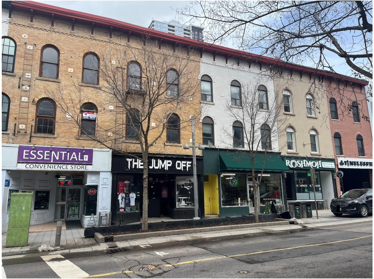
Front Façade of 8-24 King Street East.
