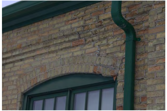
Figures 6 & 7: (left) View of north and west elevation of main factory building noting masonry repairs with red brick (right) View of "wing" addition noting original yellow/buff and red bricks throughout (MHBC, 2026).
