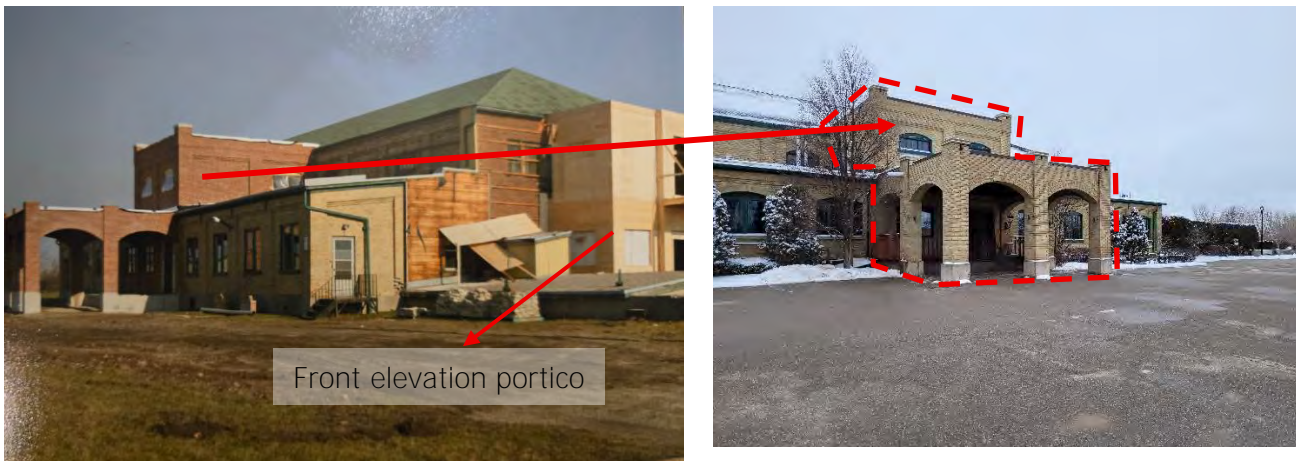
Figures 1 & 2: (left) View of construction of addition to west elevation, as well as a portion of the front elevation two storey portico (c. 2005) (right) View of existing west elevation (MHBC 2026) noting contemporary additions.
