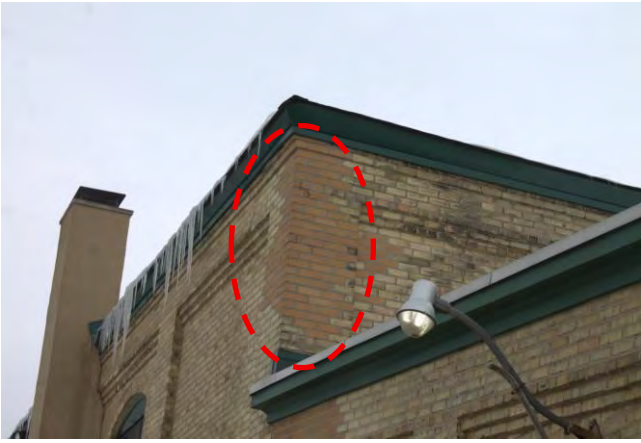
Figures 6 & 7: (left) View of north and west elevation of main factory building noting masonry repairs with red brick (right) View of "wing" addition noting original yellow/buff and red bricks throughout (MHBC, 2026).
