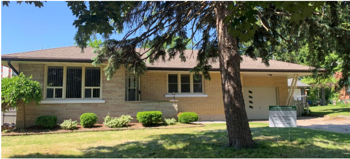
Figure 2: Front view of existing dwelling at 5 South Drive
