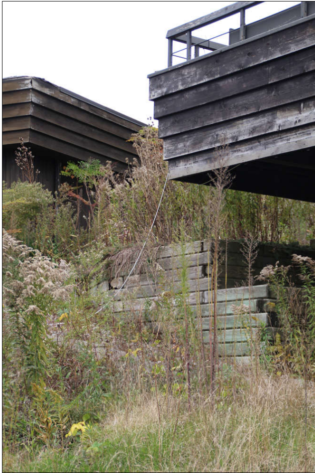
Figure 35 timber retaining wall
