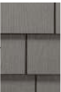
New "Shingles" - to Detailing between new windows; and - within gables of addition
