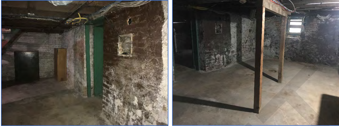
Figure 52: View of rear portion of the basement. Note the brick covered with whitewash and parging
