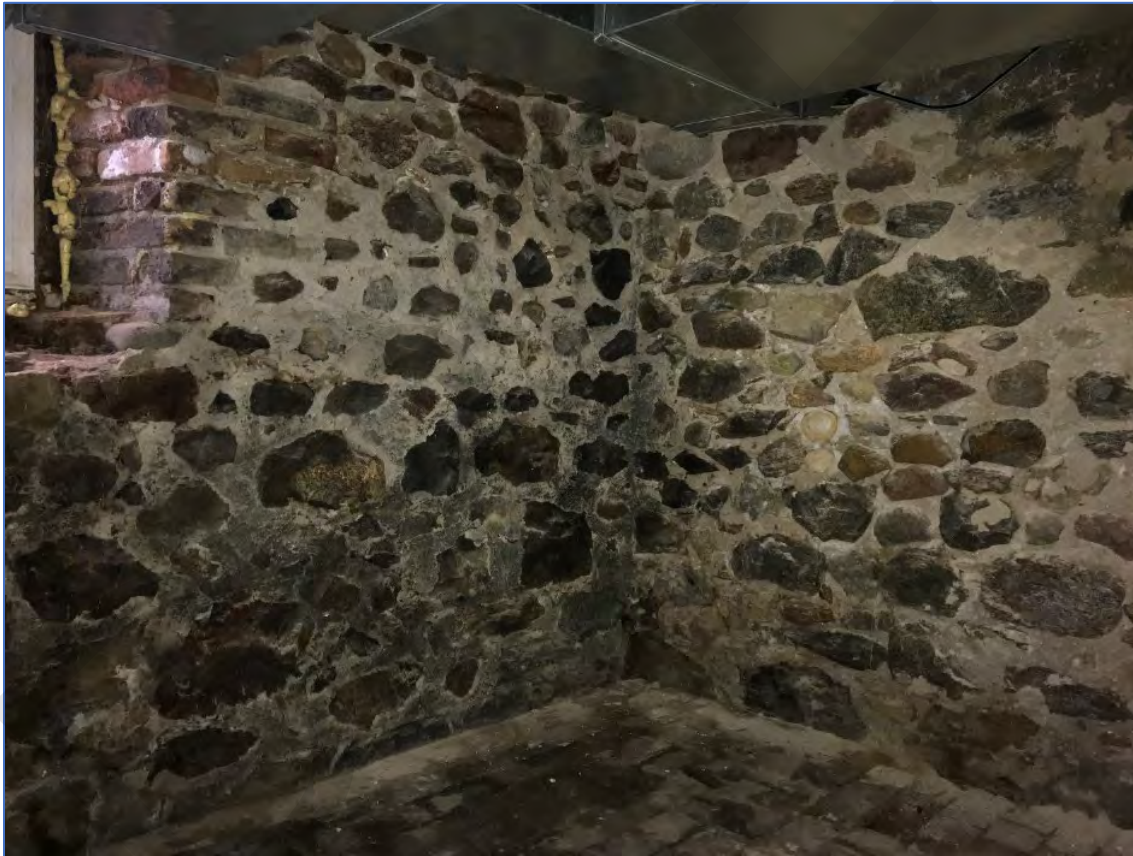
Figure 53: View of foundation wall showing mix of brick and stone walls with brick flooring
