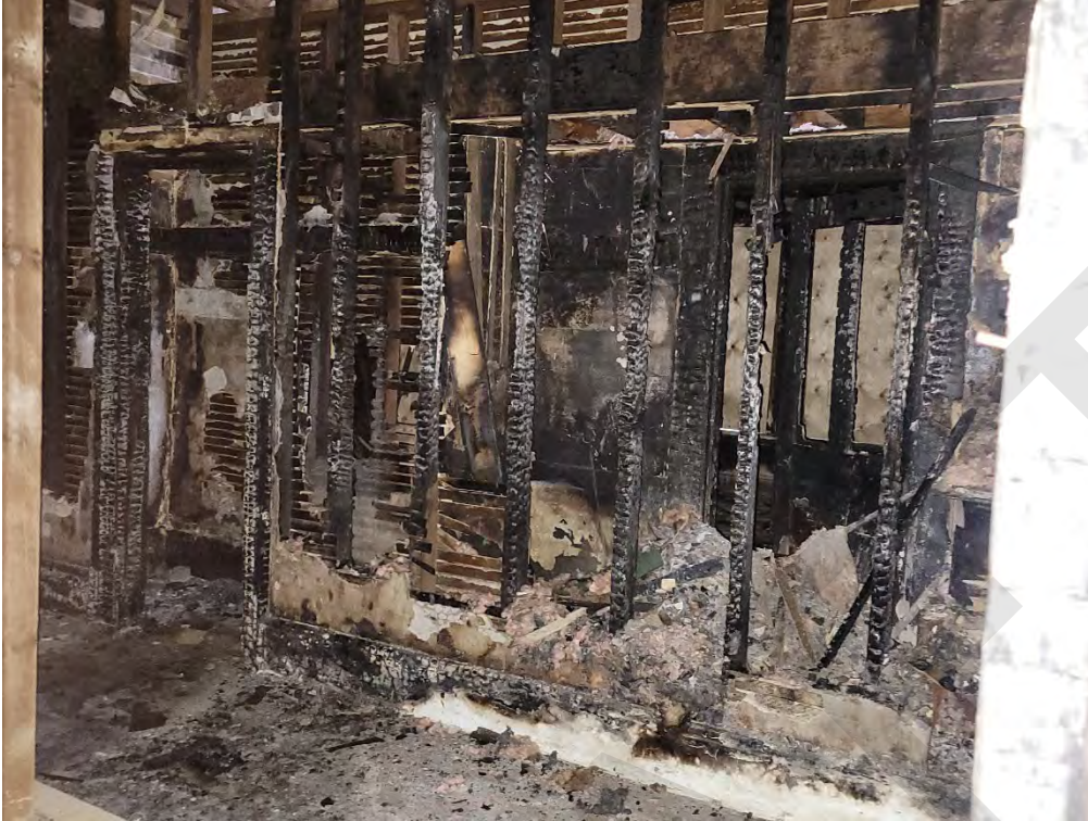
Figure 56: Fire Damage, second floor interior wall (provided by Masri O Architects)
