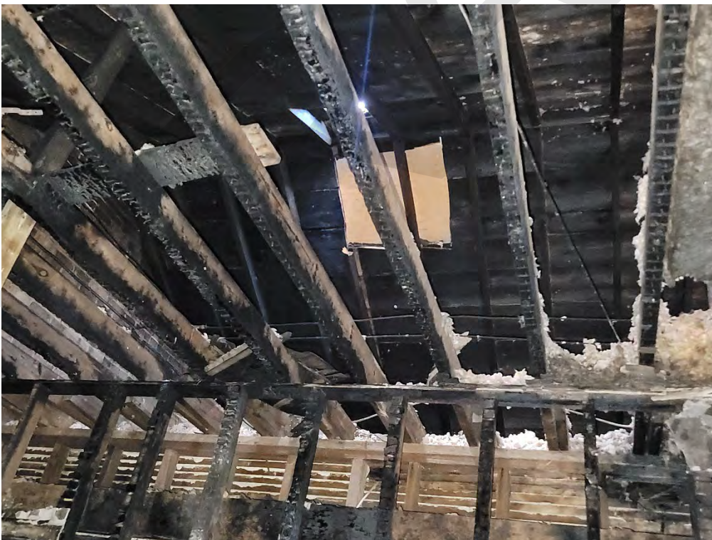
Figure 57: Fire Damage, roof from interior, second floor (provided by Masri O Architects)
