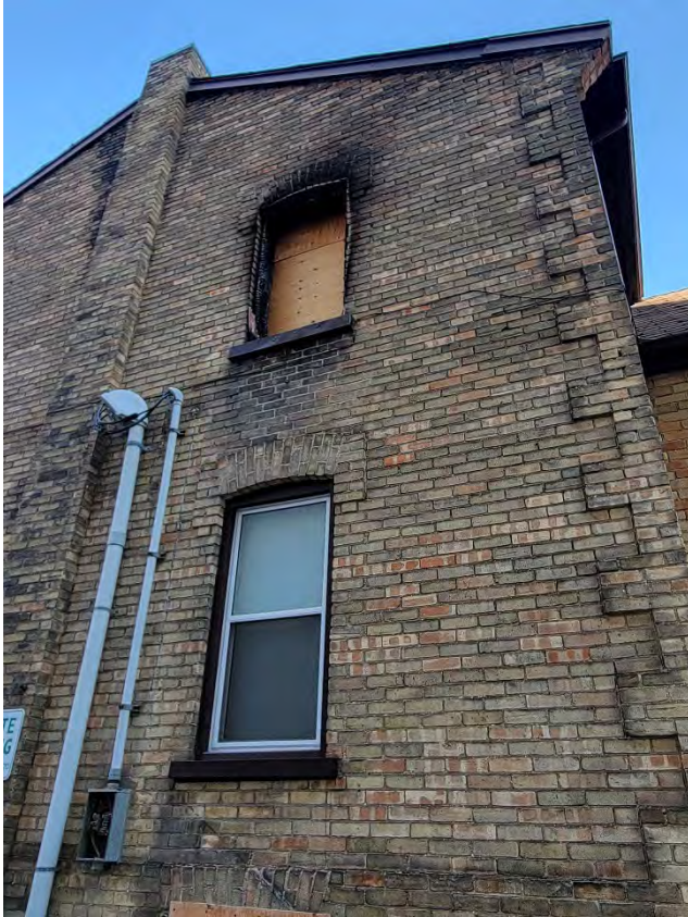
Figure 58: Fire Damage, exterior, side (south) elevation (provided by Masri O Architects)
