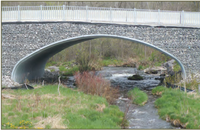
Photo 14. Arched tunnel allowing natural stream crossing. © D. Seburn
