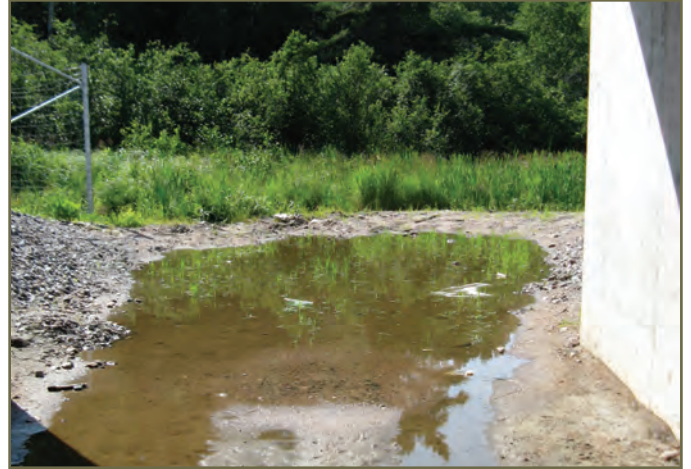
Photo 31. Water accumulation at tunnel entrance. © K. Gunson
