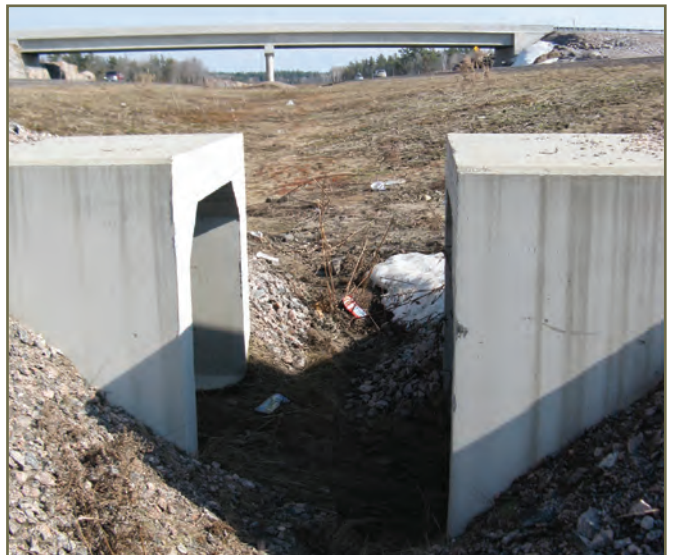
Photo 10. Box tunnels in median that should be connected with a fence when intended for wildlife passage. © K. Gunson
