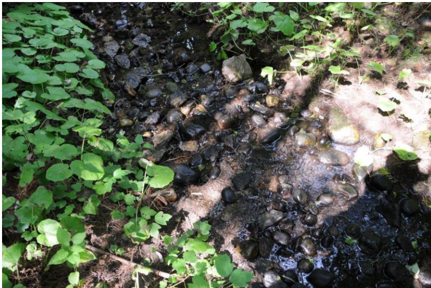
Twin 1.2 m culverts (above) with a river stone entrance apron at the headwall (below) cross under the Biehn Drive cul-de-sac and connect to a permanent Strasburg Creek tributary to the north
