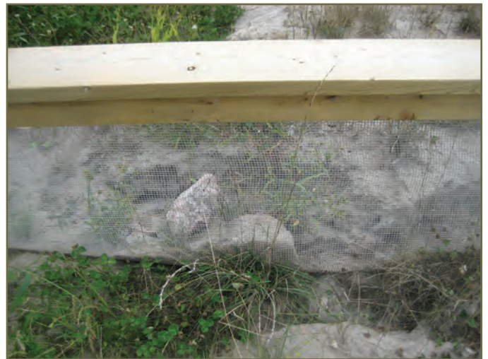
Photo 39. Hardwire cloth with 1/4 inch mesh, wood frame, and top lip © K.Gunson
