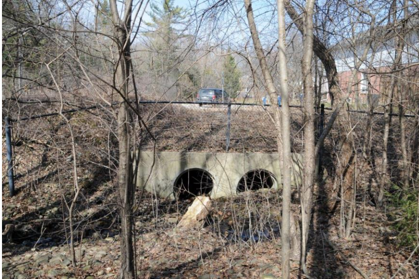
Twin 1.2 m culverts (above) with a river stone entrance apron at the headwall (below) cross under the Biehn Drive cul-de-sac and connect to a permanent Strasburg Creek tributary to the north
