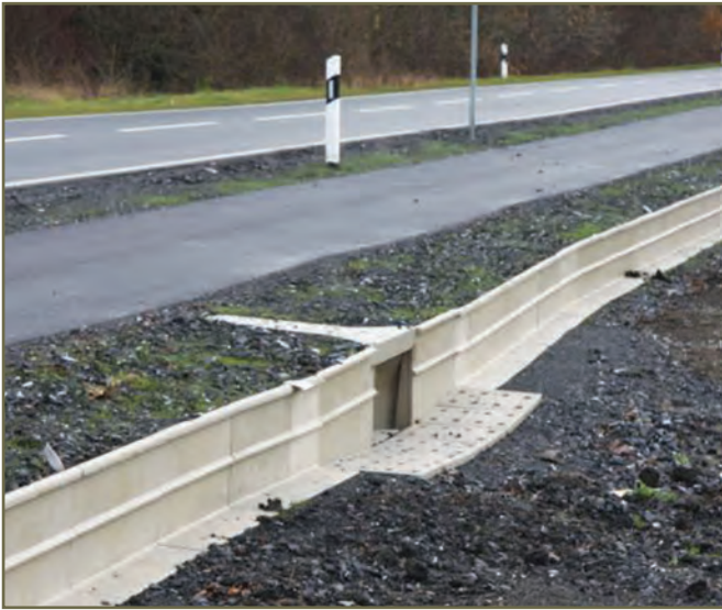
Photo 7. Open- and closed-top variation, Germany. © ACO International
