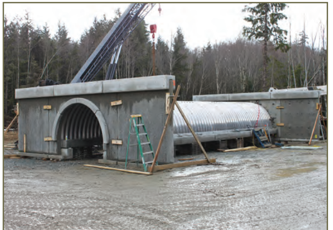
Photo 19. Arch culvert preassembled off site © K. Williams
