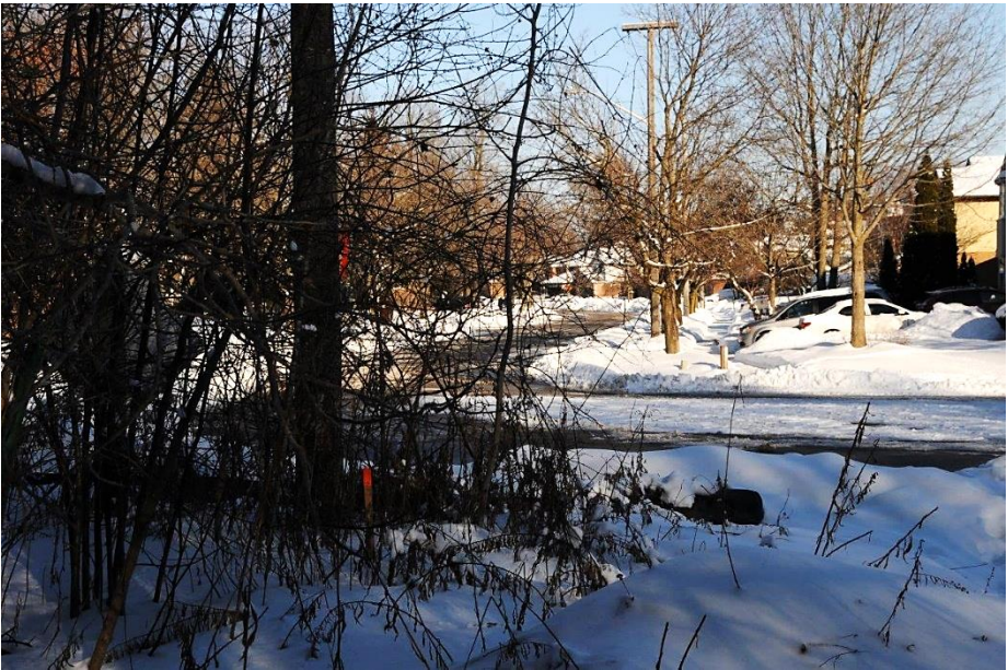
Stakes identify the roadway ROW limits (red, above) and centreline alignment (yellow, below) through the PSW at the Biehn Drive cul-de-sac
