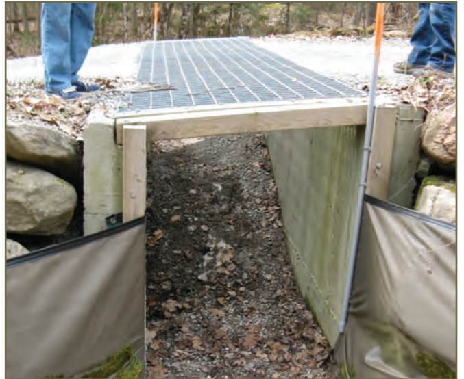
Photo 6 Open-top and open-bottom at Wild Rice Trail, Six Mile Lake. © K. Gunson
