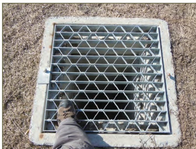
Photo 29. Zoom-in of skylight in median on Terry Fox Extension, Ottawa, Ontario. © D. Seburn
