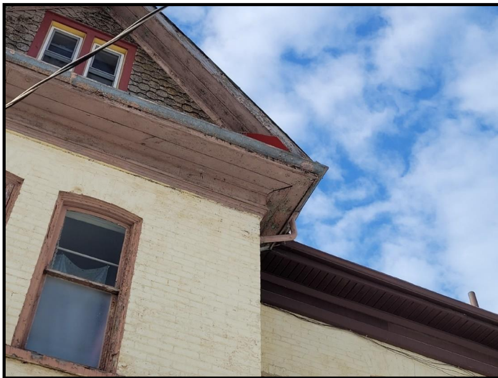
Image 18: Subject Property – Molded Wooden Cornice Showing Area Clad with Aluminium Flashing (Photo taken December 20, 2021; Facing West)
