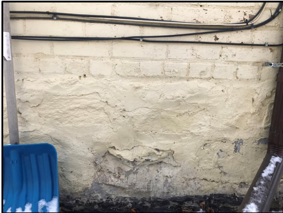
Image 38: Subject Property – Single Masonry Course Laid in Header Pattern on Foundation (Photo taken December 20, 2021; Facing South)
