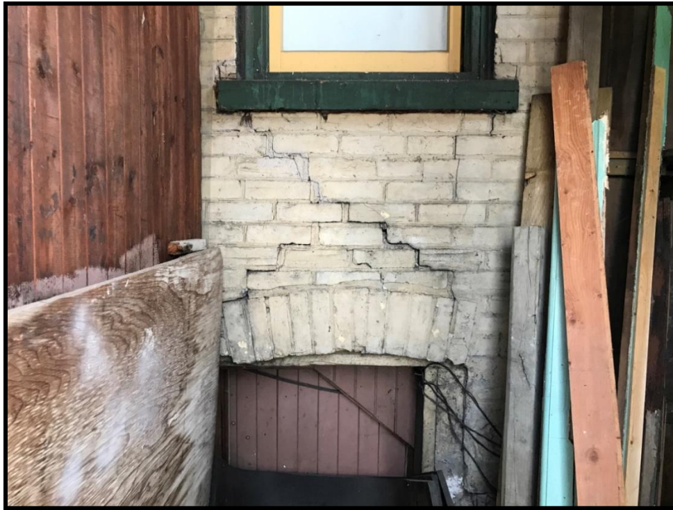
Image 29: Subject Building – Running Cracks in Masonry and Fallen Arch (Photo taken December 20, 2021; Facing Southwest)
