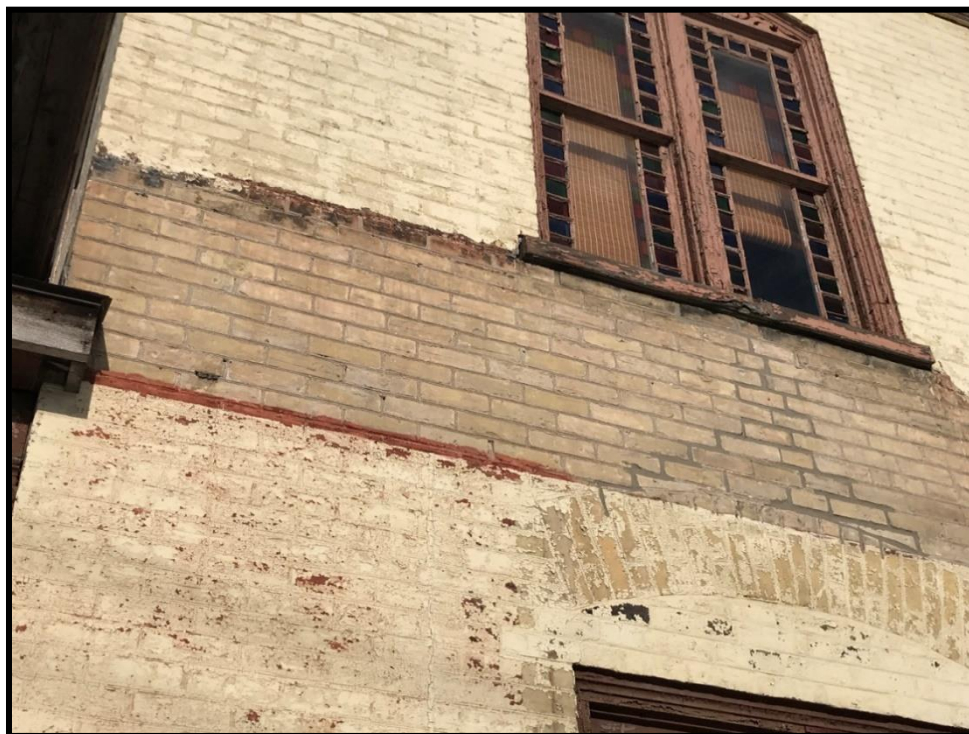
Image 10: Subject Property – Unpainted Brick Area Revealing Buff Brick Construction (Photo taken December 20, 2021; Facing North)
