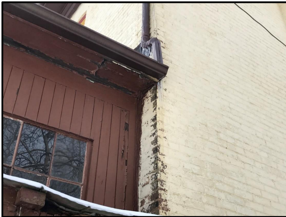
Image 32: Subject Property – Brick Discolouration Showing Water Shedding Issues (Photo taken December 20, 2021; Facing Southwest)
