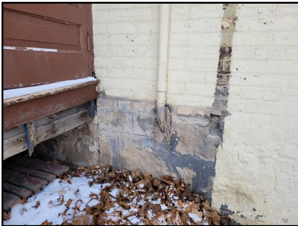
Image 20: Subject Property – Stone Foundation with Coursed Mortar Parging (Photo taken December 20, 2021; Facing Southwest)
