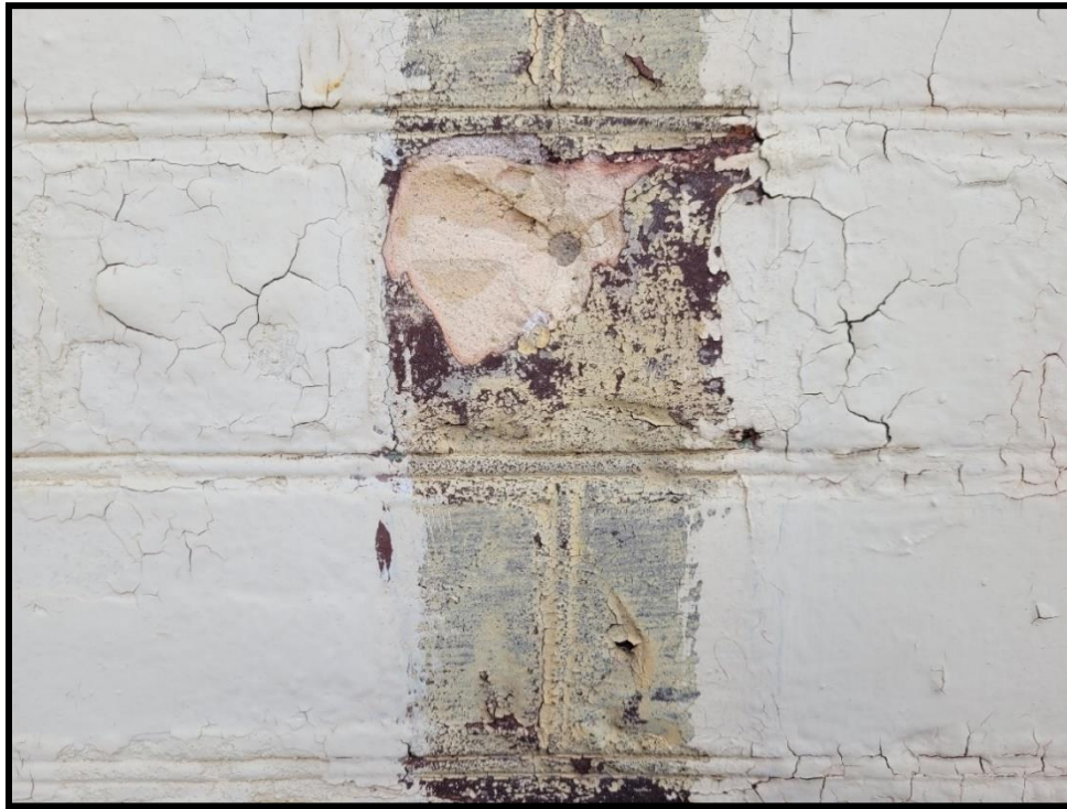
Image 21: Subject Property – Brick Detail Showing Red Glazing and Beaded Mortar Profile (Photo taken December 20, 2021; Facing Southwest)
