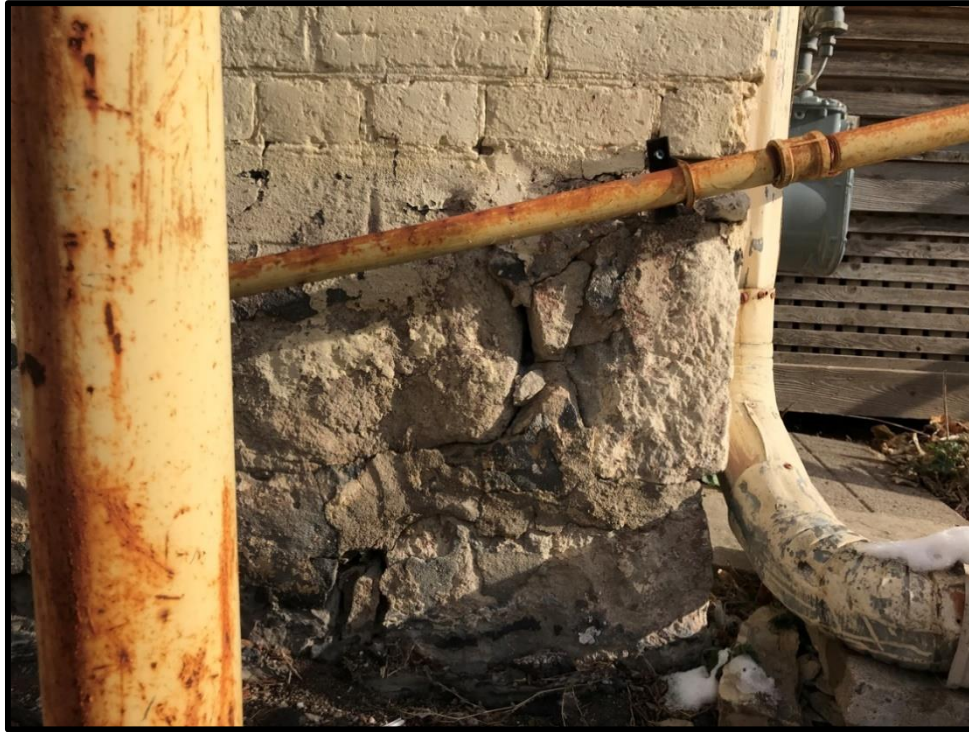
Image 49: Subject Property – Stone Foundation with Deteriorated Mortar (Photo taken December 20, 2021; Facing East)
