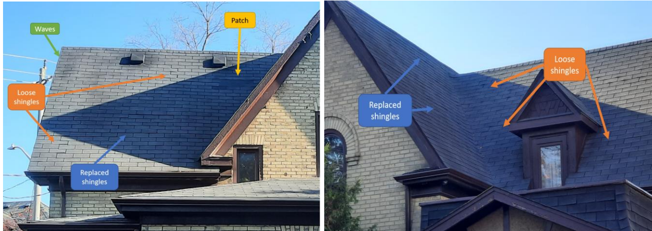
Figure 2-3: Existing Condition of Roof (Rear and Front Views)
