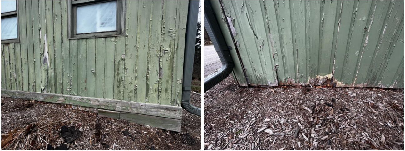
Figure 4-5: Deterioration of the Existing Sunroom
