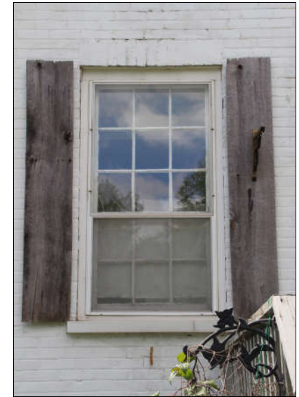
Figure 21 9/6 window, 1874 section
