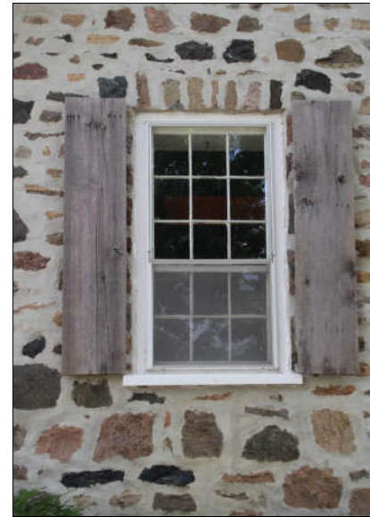
Figure 20 9/6 window, 1864 section
