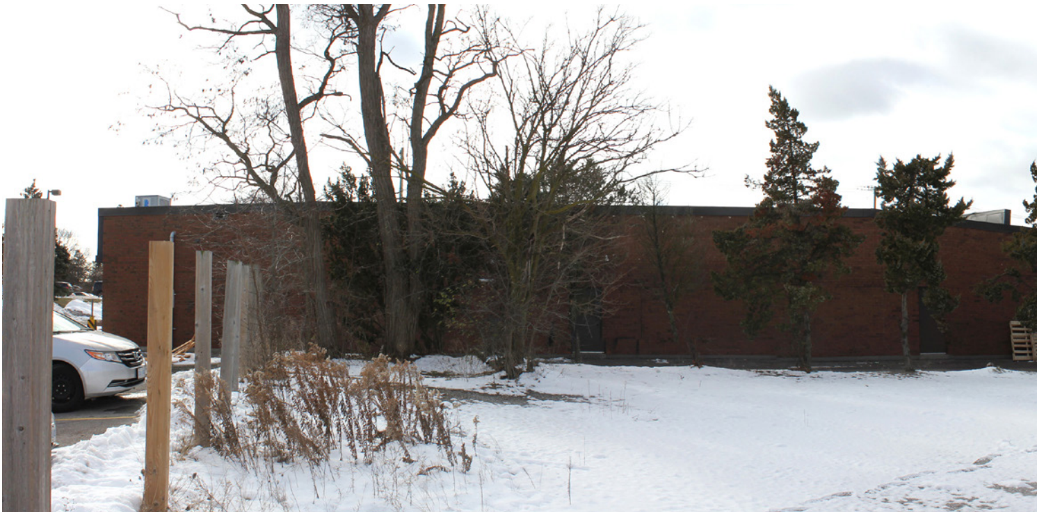
View looking from north-east side of the Site at 25 Sportsworld Drive.
