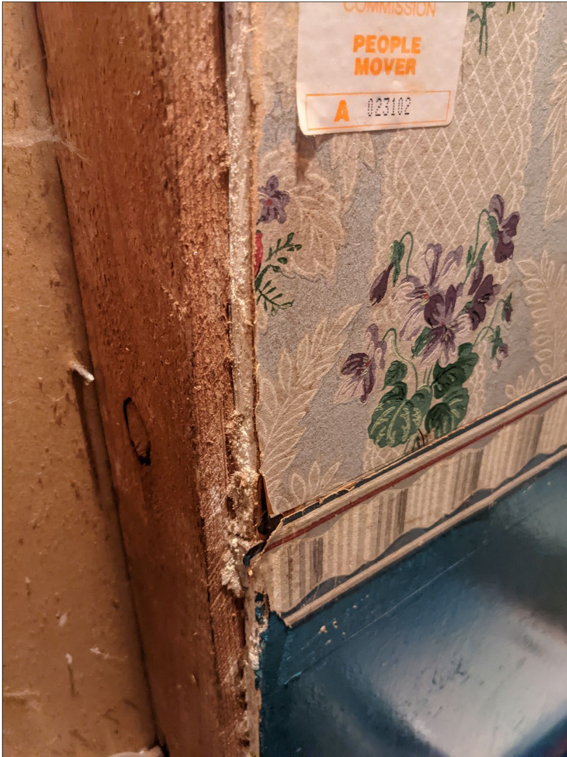
Figure 25: Photograph of interior composition of the house showing conventional studs (Tacoma Engineers Ltd., 2022).
