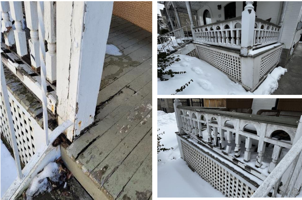
Figures 3-5: Deterioration of Existing Porch
