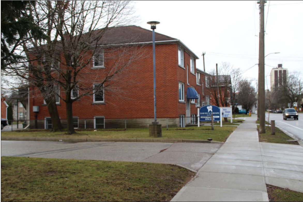
Figure 20 office-residential six-plexes on Frederick Street, west side of subject property
