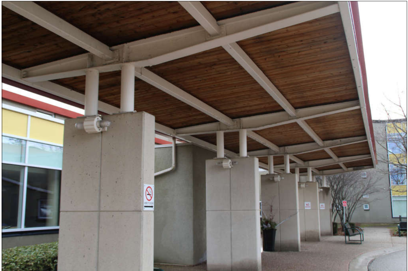
Figure 38 entry canopy The 1-storey administration wing has a clerestory (Figure 40) with large windows placed at the upper level on the east side to provide light and glazing throughout the lower walls on the west and part of the north side, providing views of the landscape (Figures 39 & 41). The ceiling exposes the metal batten roof and is supported by large concrete columns (Figure 40).
