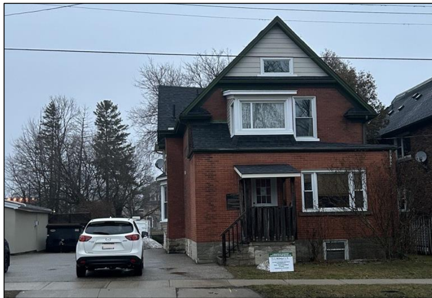
Figure 2: Front view of the existing site
