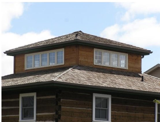
Detail of the pyramidal cedar shingle roof, pine fascia and frieze and glass roof lantern with prefinished metal covered wood windows with muntins
