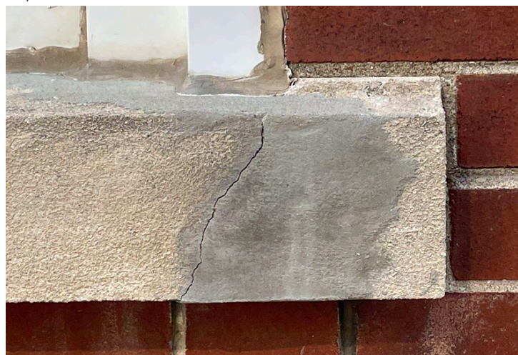
Figure 13. Cracking and deterioration in the sill. The repair is visually intrusive and measures should be taken to rehabilitate the sill to make it visually compatible to its original design. This inspection was undertaken with the naked eye and is not intended to identify any structural issues. (Source: mCs, July 2021)
