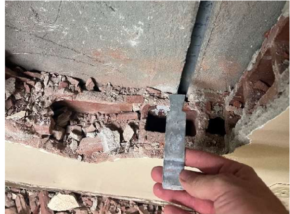
Fig 6: Looking down at opening, dovetail anchor
