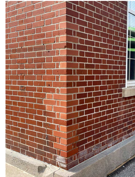
Figure 11. Detail of the Queen Street Facade (left) and right side of the rear facade (right) showing locations where efflorescence and mortar deterioration has occurred due to water damage. (Source: mCs, July 2021)
