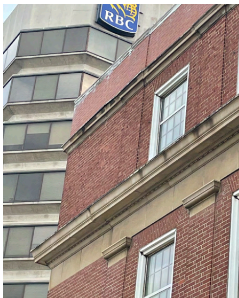
Figure 9. Detail of the front facade fronting Duke Street West. The parapet brick appears to have been replaced as variation in brick stain was observed. (Source: mCs, July 2021)
