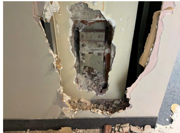
Fig 2: Typical column splice, above 2 nd floor
