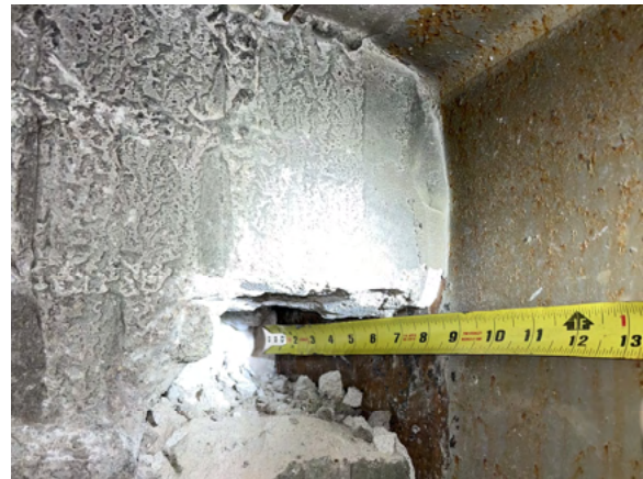
Fig 4: Typical beam bearing length on exterior wall
