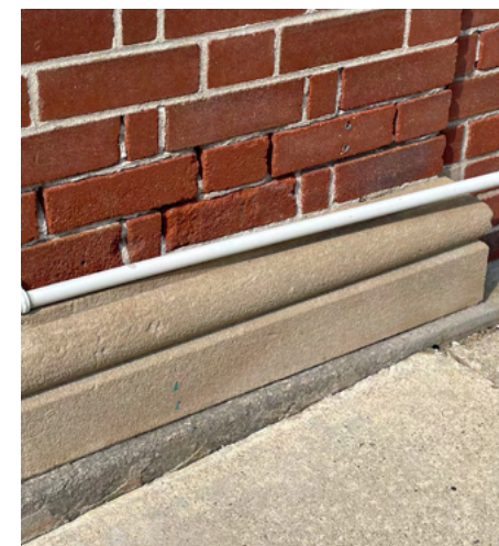
Figure 14. Poor repairs to masonry and mortar. Bricks should be repointed with mortar that is compatible with existing. (Source: mCs, July 2021)
