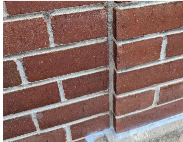
Fig 12: Typical continuous vertical joint at brick pier
