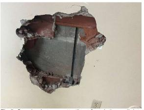
Fig 5: Opening in terra cotta tile at foundation wall, interior
