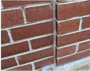
Fig 12: Typical continuous vertical joint at brick pier
