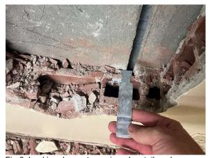
Fig 6: Looking down at opening, dovetail anchor
