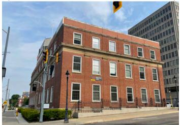
Figure 12. Perspective View of the subject property from Duke St W and Queen St intersection showing the heritage attributes of the building: 11 bays along Duke and 6 bays along Queen, the concrete band between the 2nd and 3rd floors, the parapet at the roofline with red brick on all facades.(Source: mCs, July 2021)
