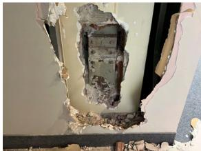
Fig 2: Typical column splice, above 2<sup>nd</sup> floor
