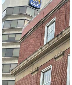
Figure 9. Detail of the front facade fronting Duke Street West. The parapet brick appears to have been replaced as variation in brick stain was observed. (Source: mCs, July 2021)
