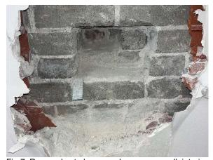
Fig 7: Removals at above-grade masonry wall, interior
